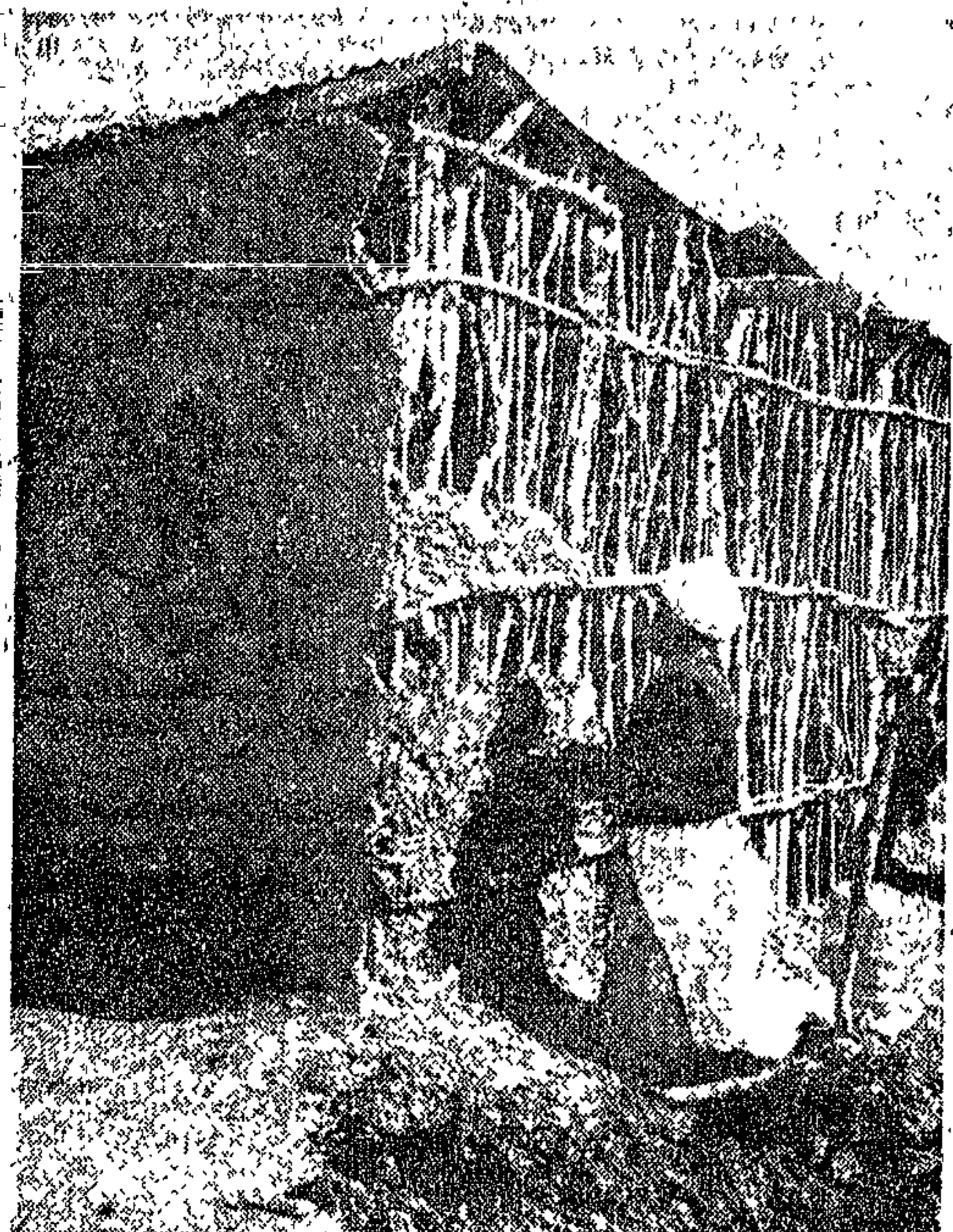
A wattle-and-daub home under construction at Heaton Trust Farm.
