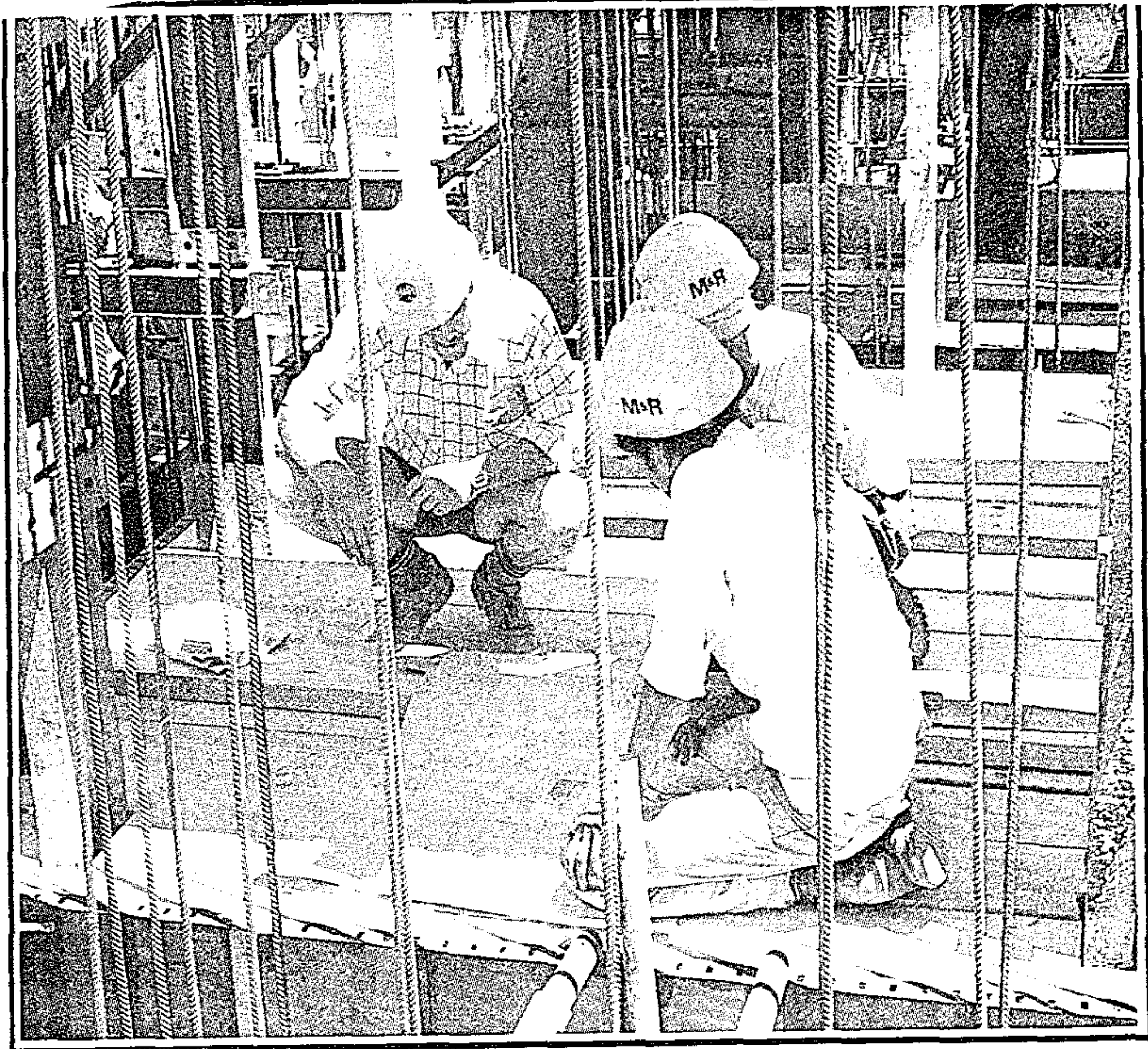
● A Murray and Roberts Buildings foreman explaining drawings to artisans on site at St John's Place.
