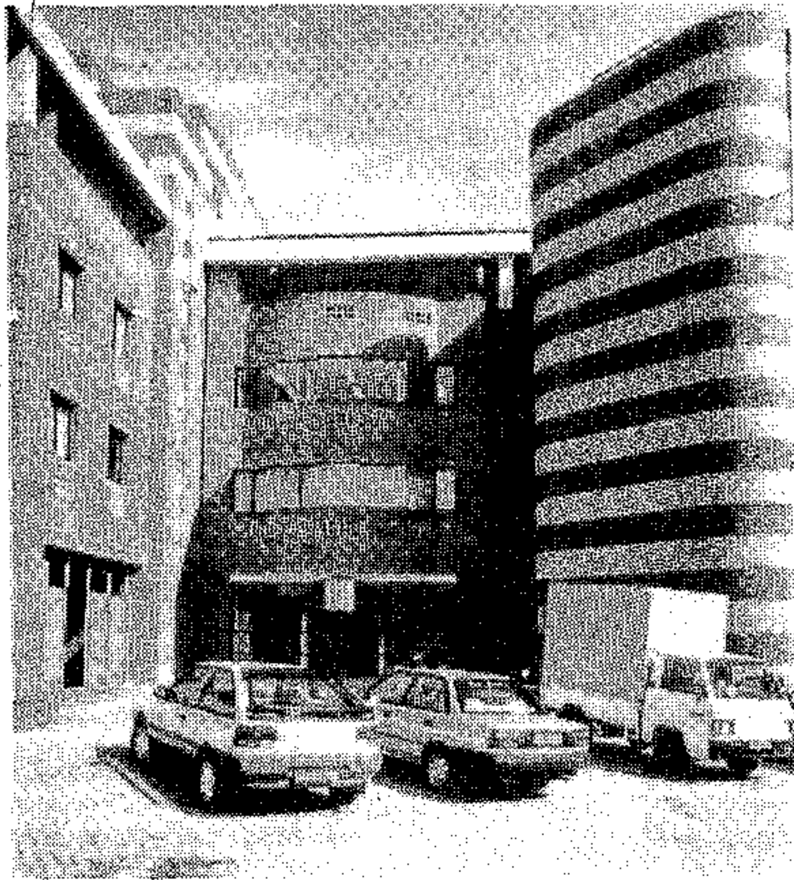
Mobil House, corner St Andrew's Road and St David's Place
