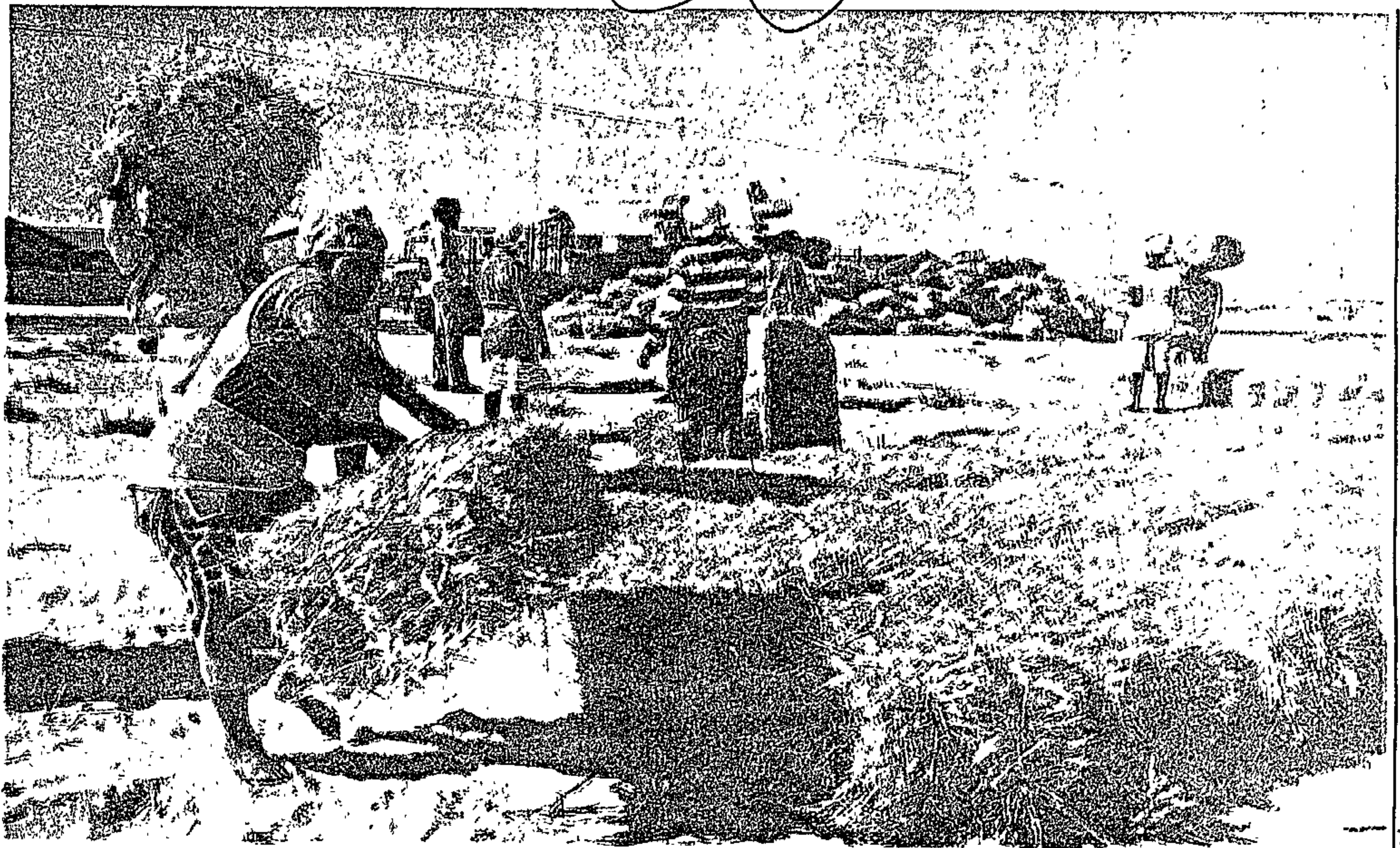
KHAYELITSHA WALL . . . Casual labourers were yesterday hired to stack a kilometre-long, double wall of straw bales along Spine Road, Khayelitsha, in a bid to stop the encroachment of thousands of tons of windswept sand from nearby construction sites. Picture: ANNE LAING
