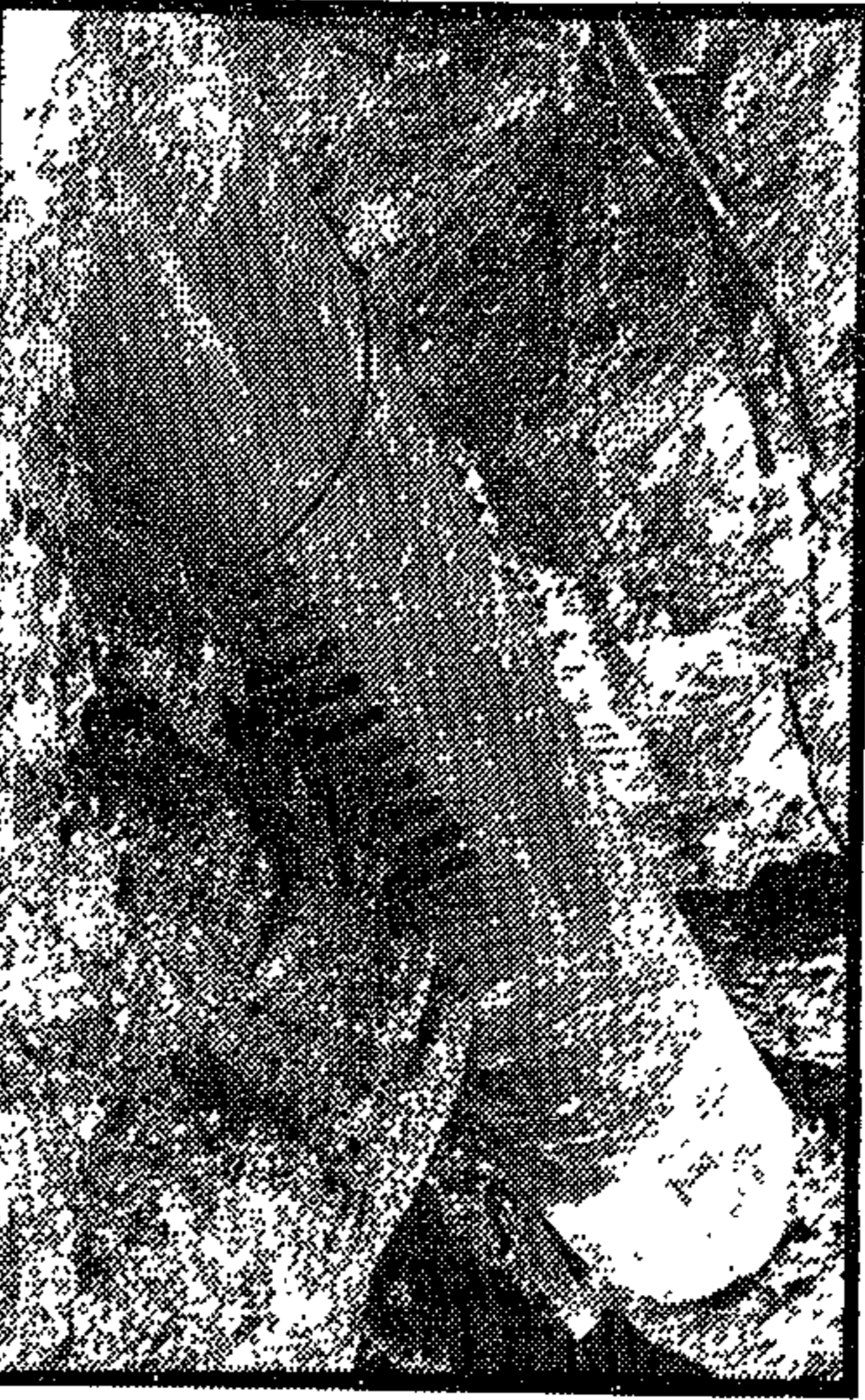
FROM left: ■ The SAICCOR factory at the head of the estuary of the Umkomaas River. ■ The fractured section of the pipe was mended with a sleeve. ■ Parks Board representative Cedrick Coetzee found the fish's gills were clogged with sludge. ■ "Where have all the fish gone," asks fisherman Cook Janssens
