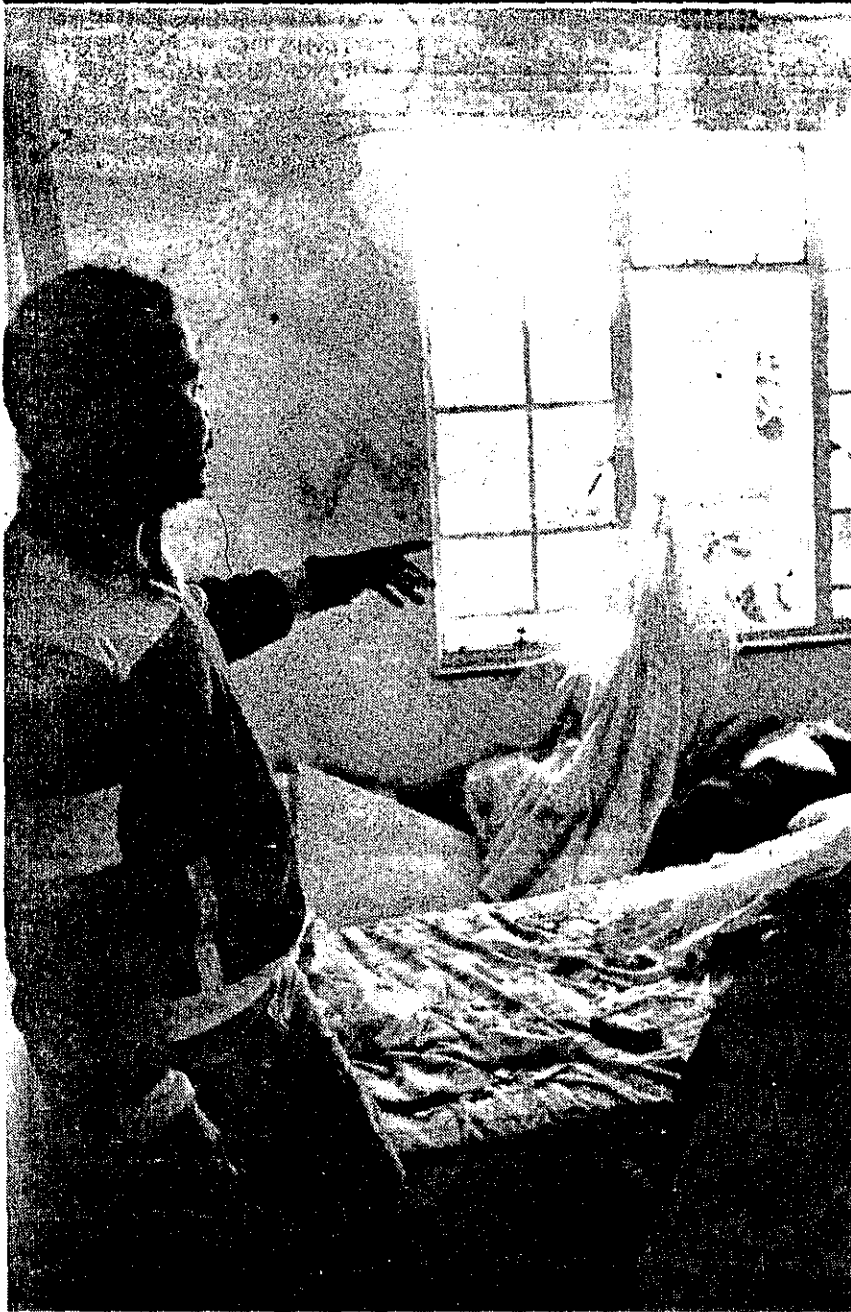
Mr SIPHIWE Thusi, a member of the Soweto Youth Congress, next to the wall which crumbled after a powerful explosion rocked the home of an activist in Klipspruit West yesterday.
