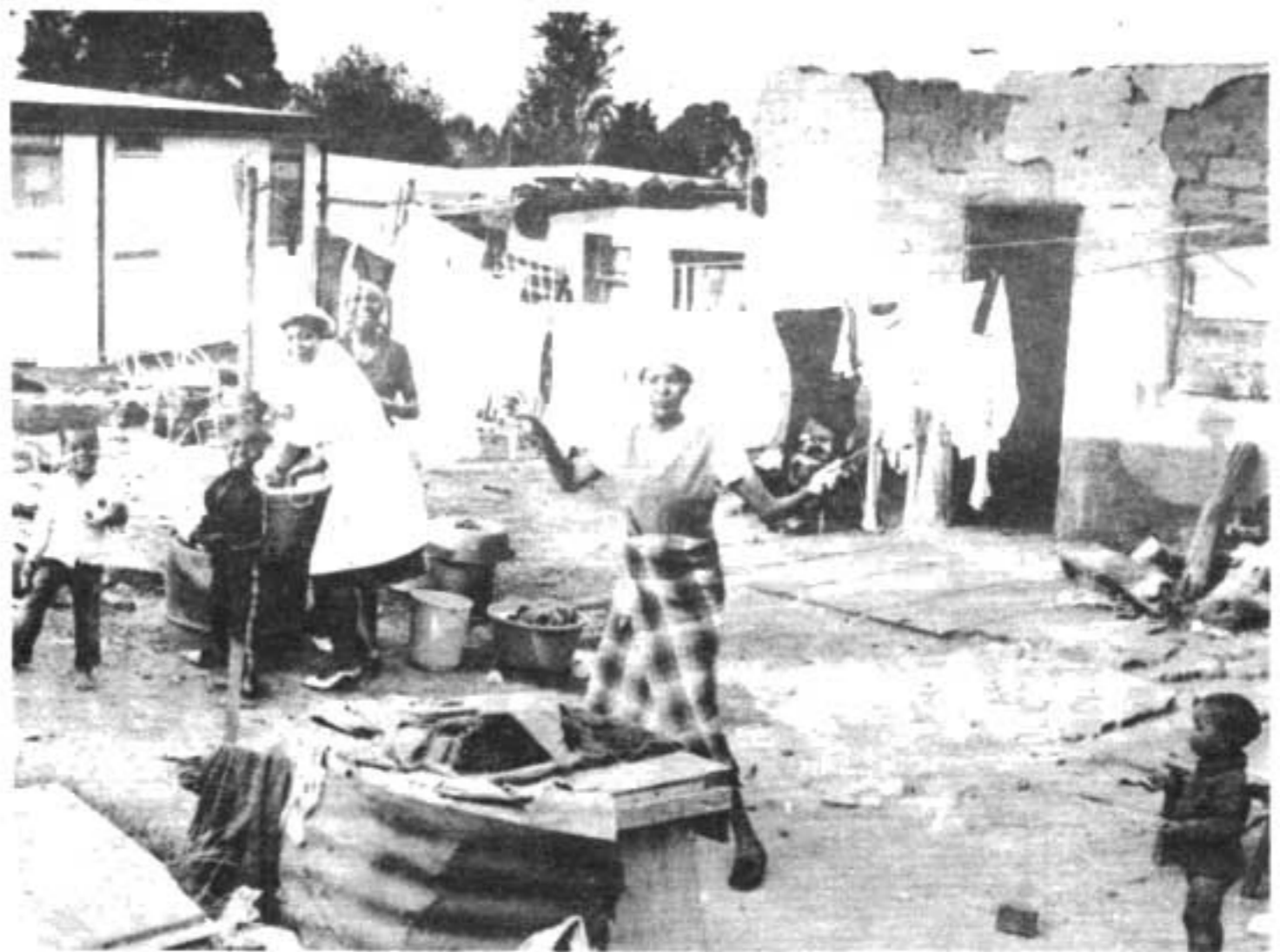
Old homes in Alexandra are demolished to make way for "redevelopment". Yet many residents say they will not be able to afford the new houses.
