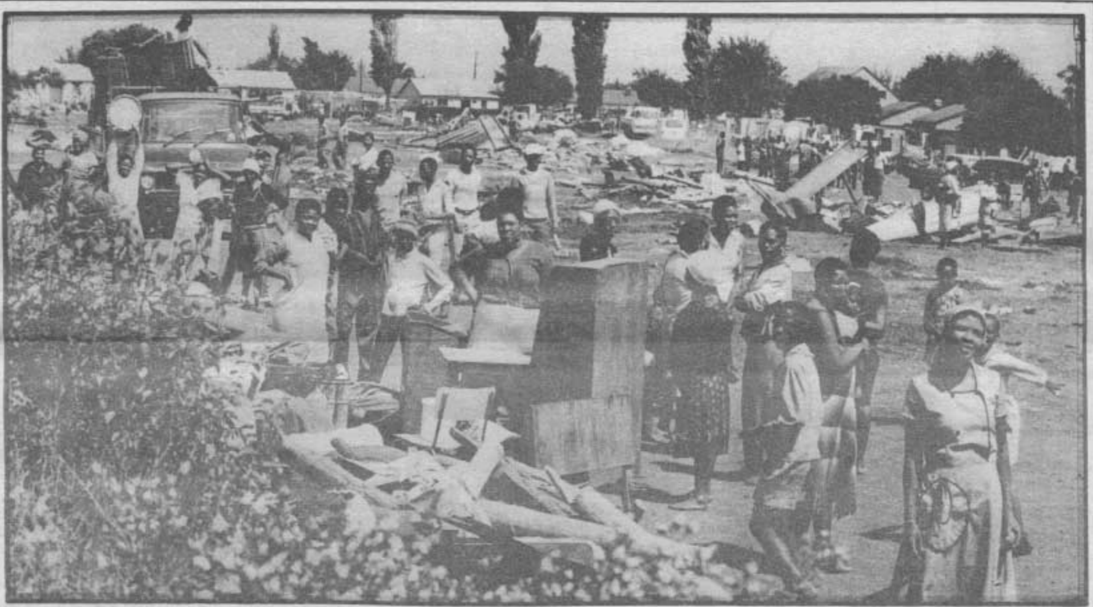
FOR thousands around the country the future is uncertain. Magopa, Leandra, Ennerdale, Huhudi, Alexandra, Katlehong, Crossroads, Badplaas, Driefontein and Soweto are just some areas where people face shack demolitions and forced removals. Piet Koornhof's directive to the Soweto Town Council that no shacks be demolished until after the festive period was at best . . . sick. Rather than saving him from world wide condemnation, Koornhof's total disregard for people to have a right to a roof over their heads was confirmed.
