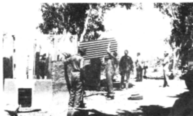
Despite the severe housing shortage, officials are constantly tearing down shacks.
