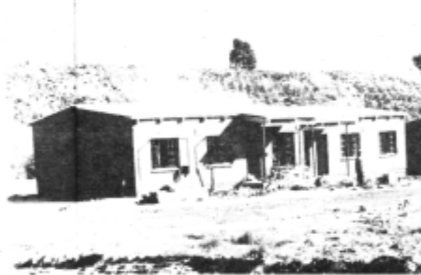
Under the new policy, the government will no longer build houses for people
