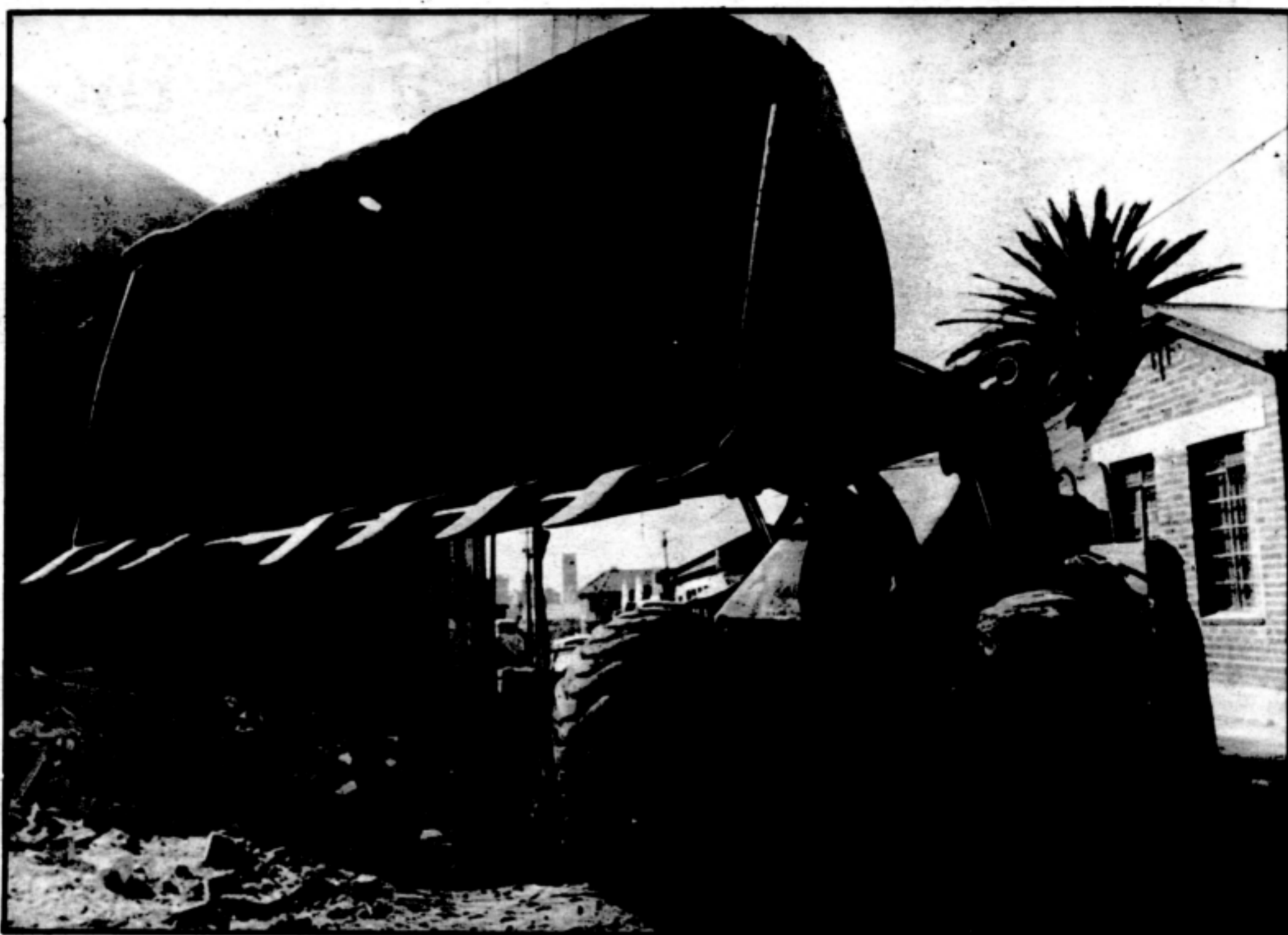
Iron jaws of a house-eating monster ... a state bulldozer in Pageview
