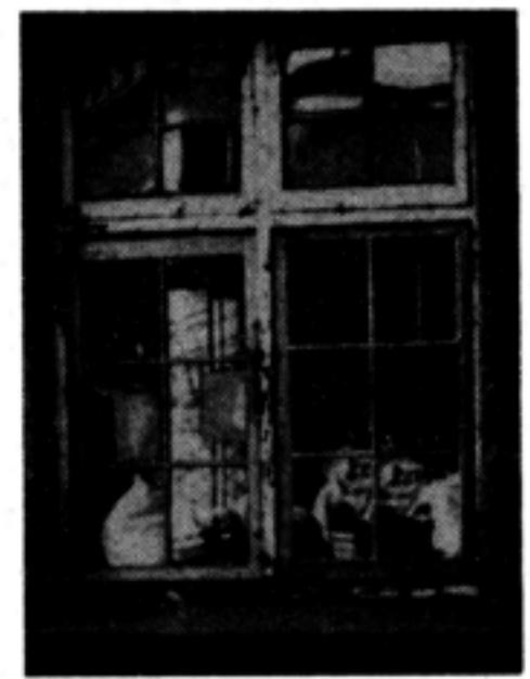
One of the windows that was NOT fixed with R5 000 00
