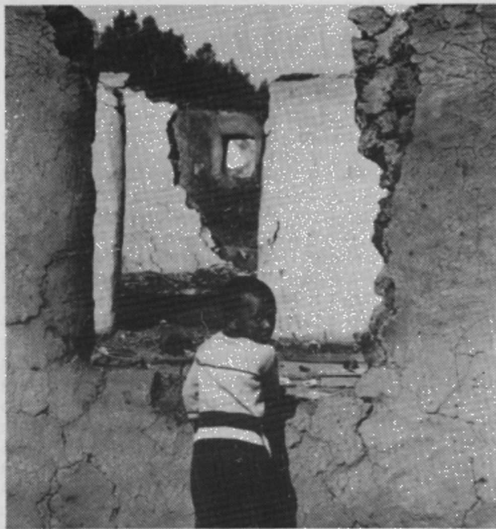
A small boy surveys the remains of his home after a veld fire
