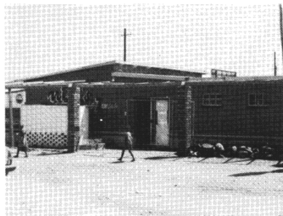
A local businessman having extended his drycleaning business has now been informed that he will have to demolish the extensions
