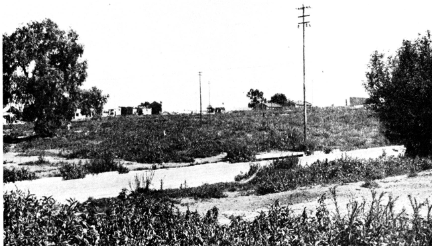
Eastern portion of Sophiatown ready for redevelopment.
