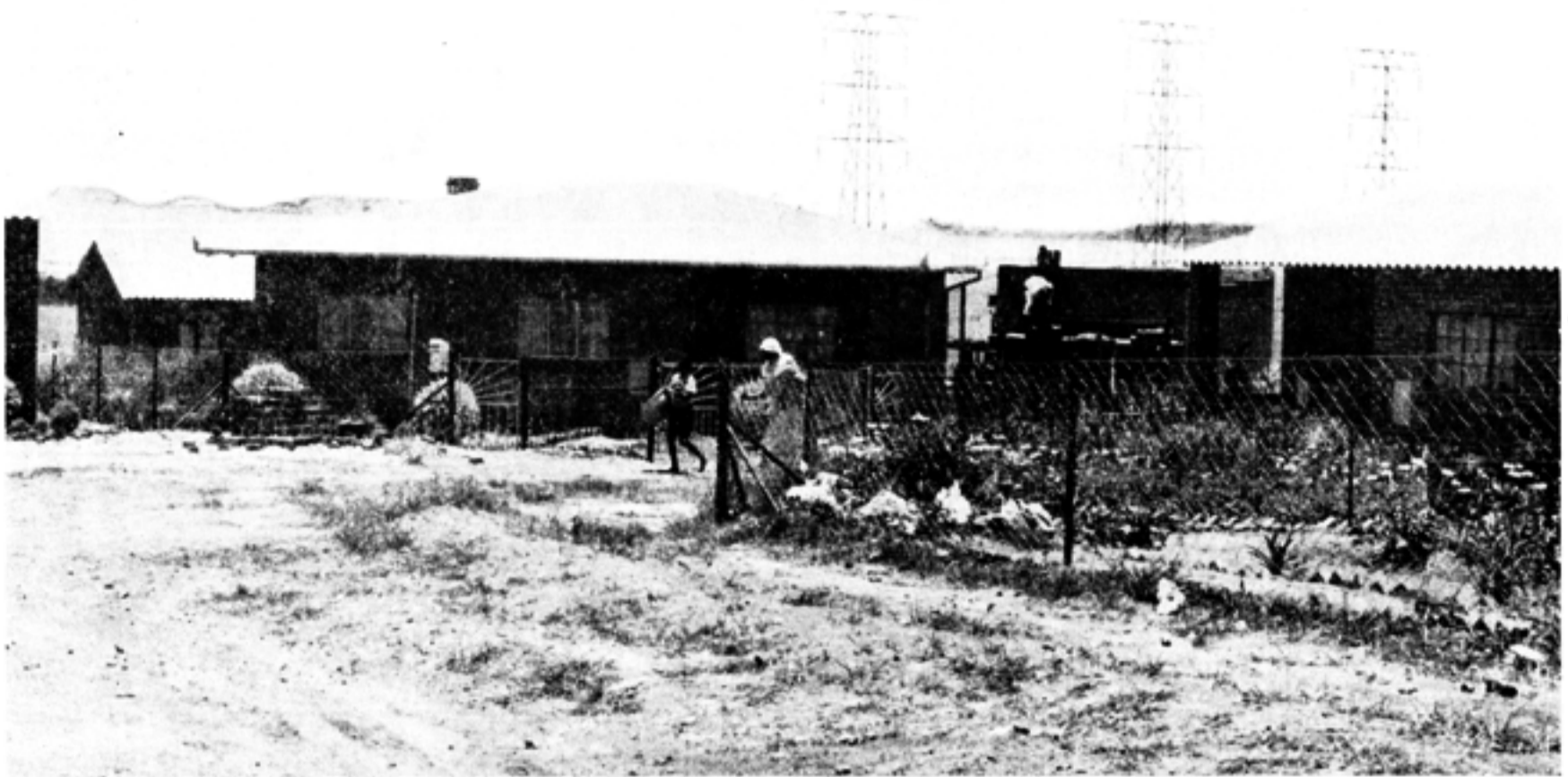
House-owner in Diepkloof erecting approved outbuilding.
