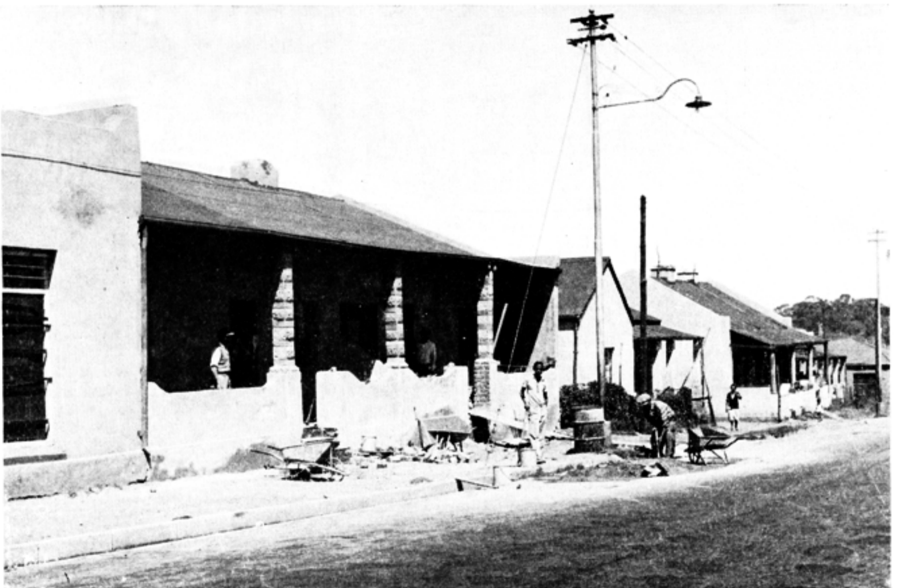
House in Newclare being renovated for occupation by Coloureds after removal of Natives.
