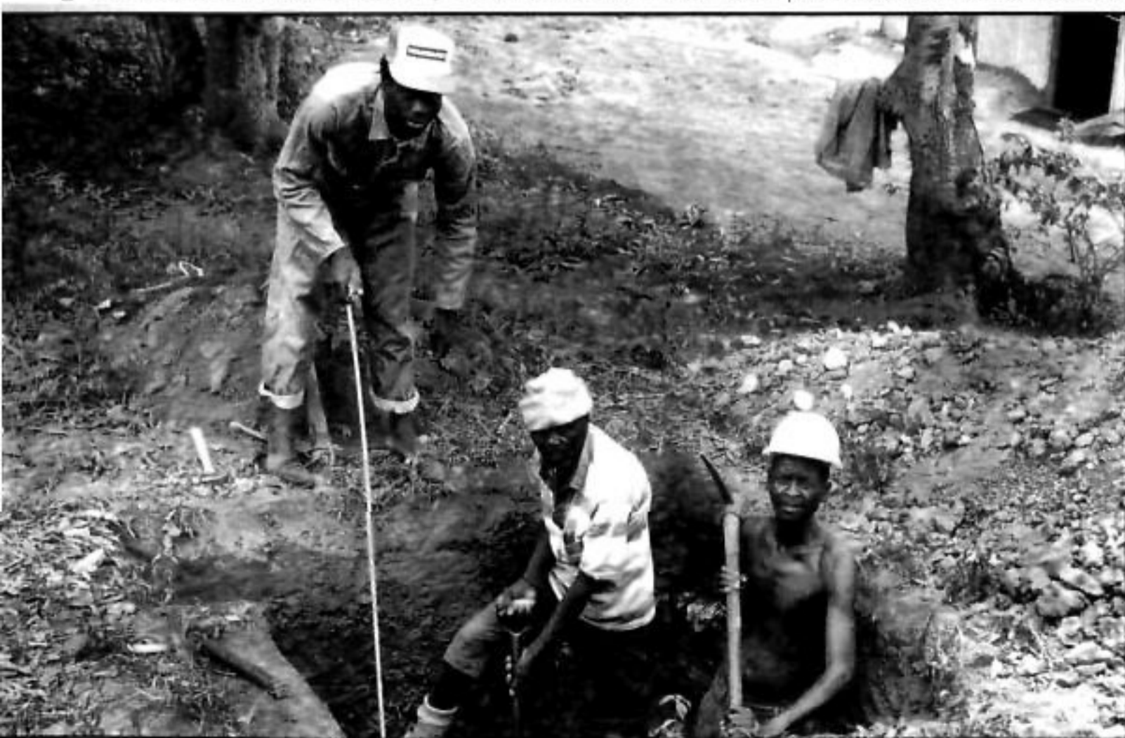
Work in progress: Zilweleni residents build their own toilets
