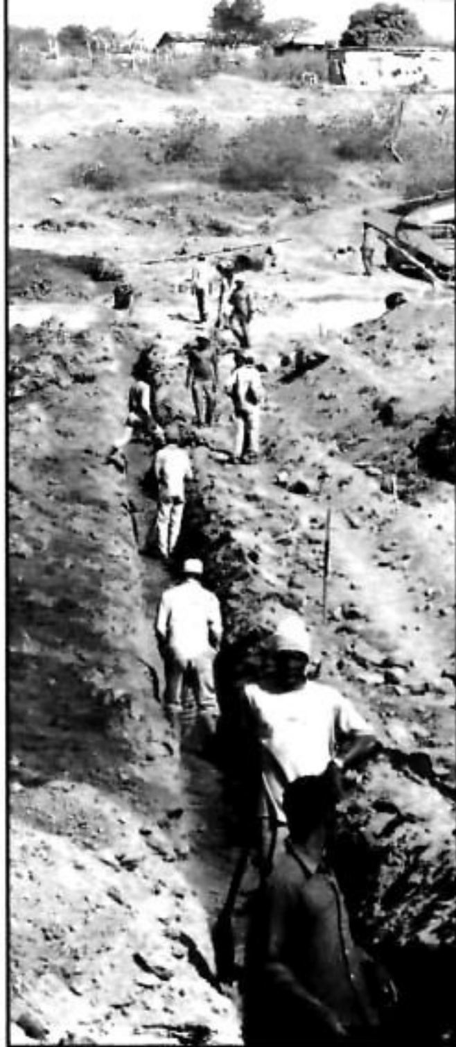
Locals lay down water pipes
