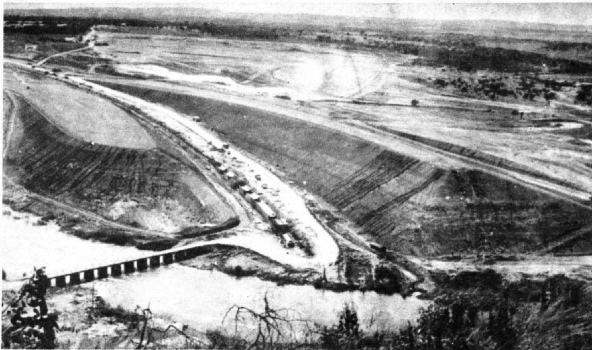
A general view of the Gove dam which Portugal is building on the Cunene in southern Angola
