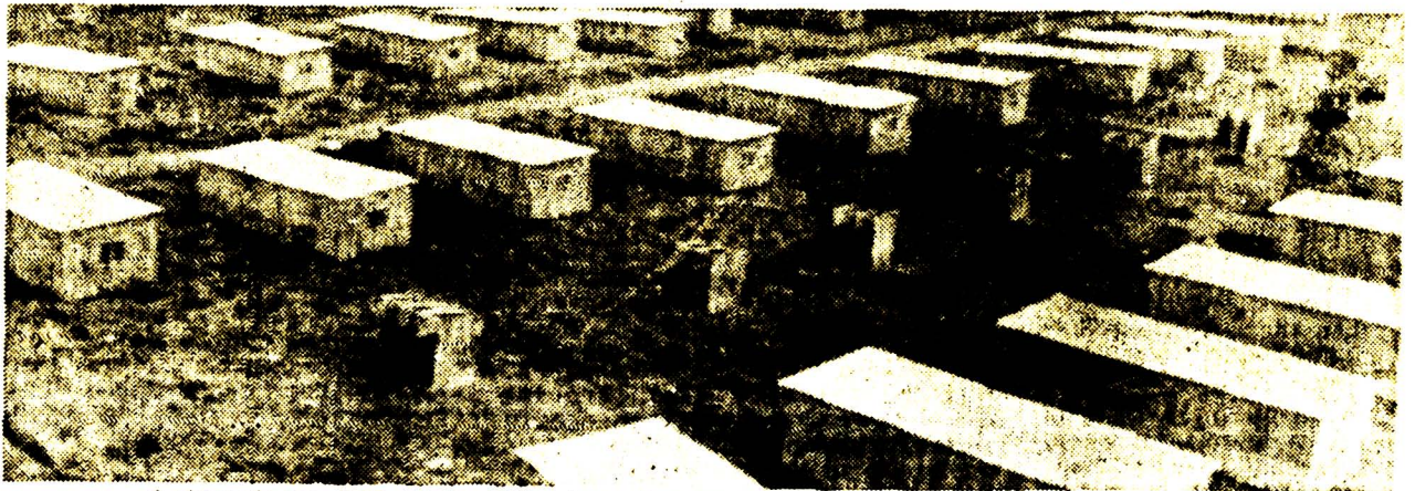
A view of part of Glenmore, 40 km from Grahamstown, showing the temporary timber-and-concrete houses built for Kenton and Klipfontein families.
