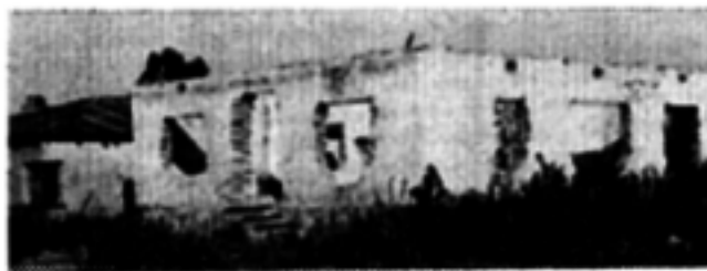
The demolished house.
