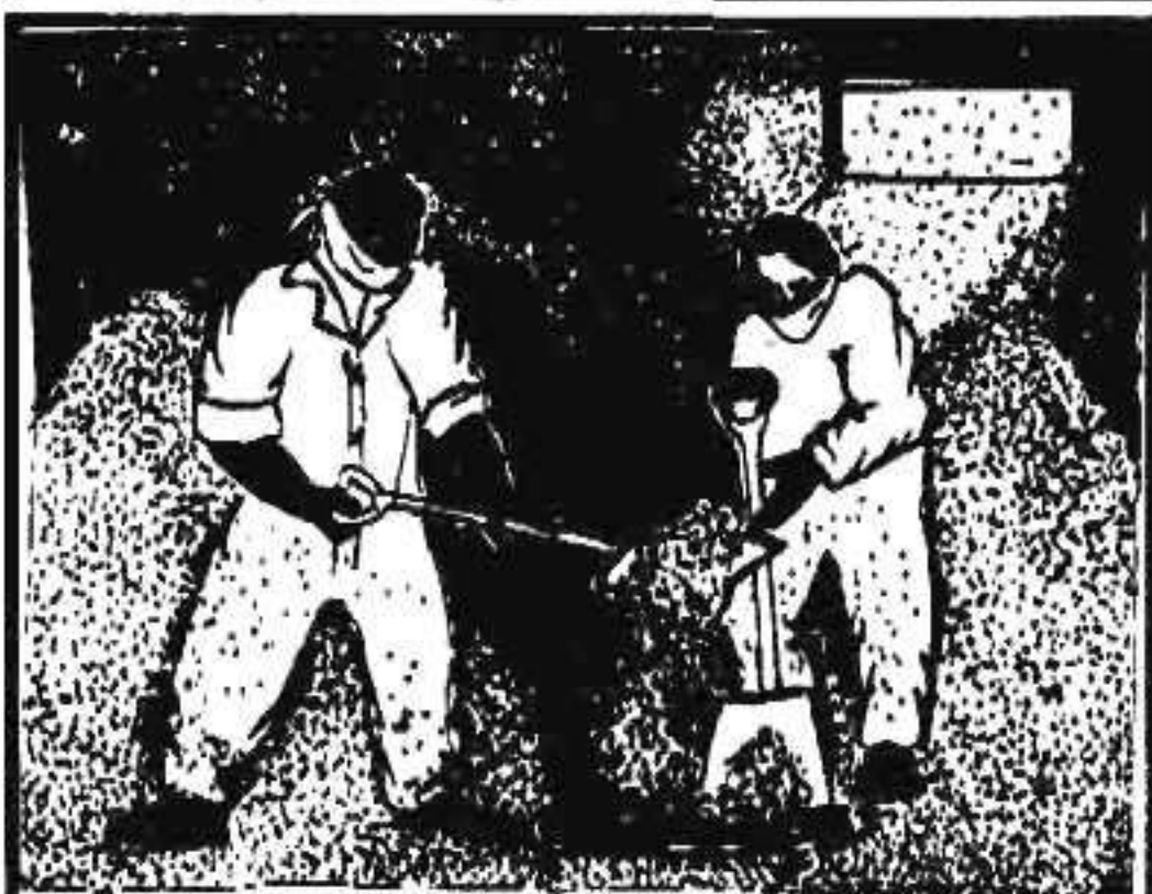
Bulk feed offloading
