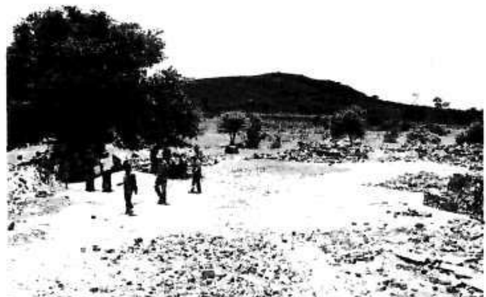
A lunch rest during the mammoth stone-cleaning operation: chipping concrete from the stones of the demolished building
