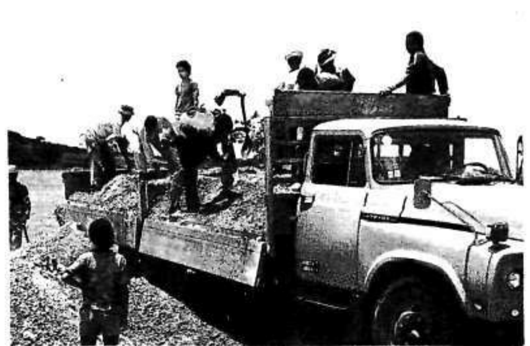
Volunteers offload building material from a SAVS truck
