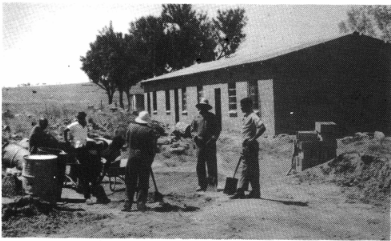
The community has started to rebuild the school at Roosboom.
