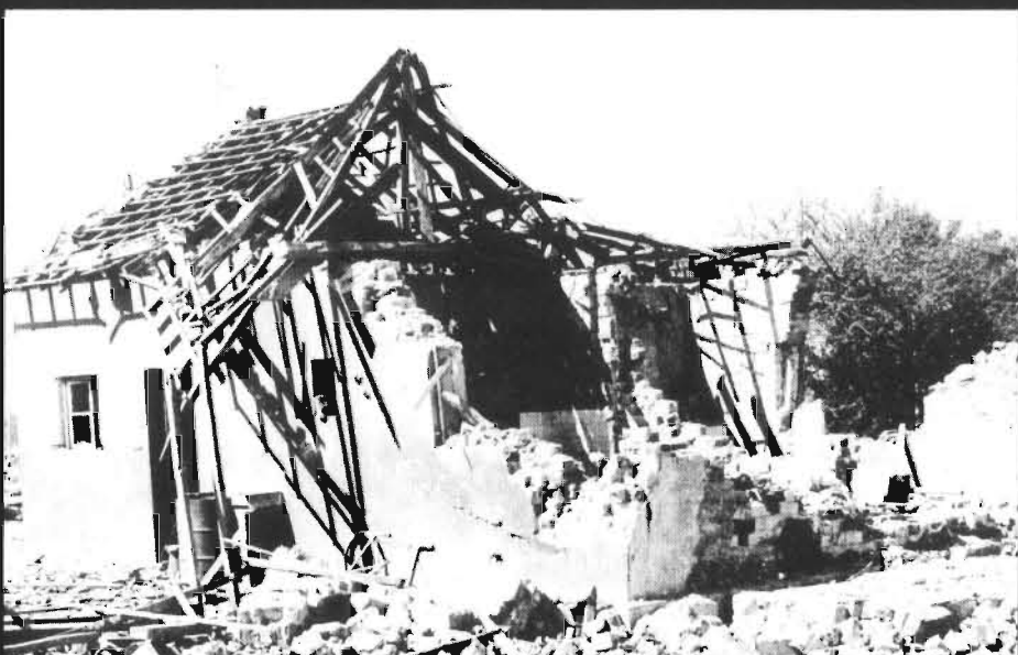
▲ On the front line: clinic at Cahama destroyed by aerial attack
