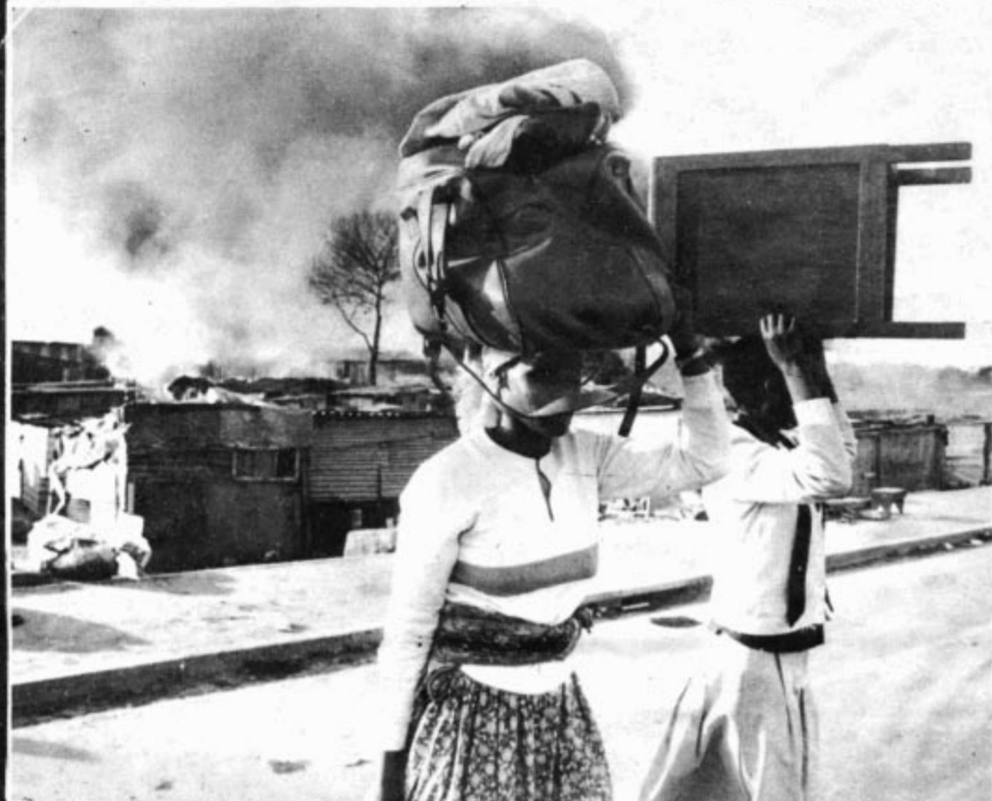
Residents trek with their belongings down Lansdowne Road as the Portland Cement Works camp burns (More pictures and reports pages 4 and 5)
