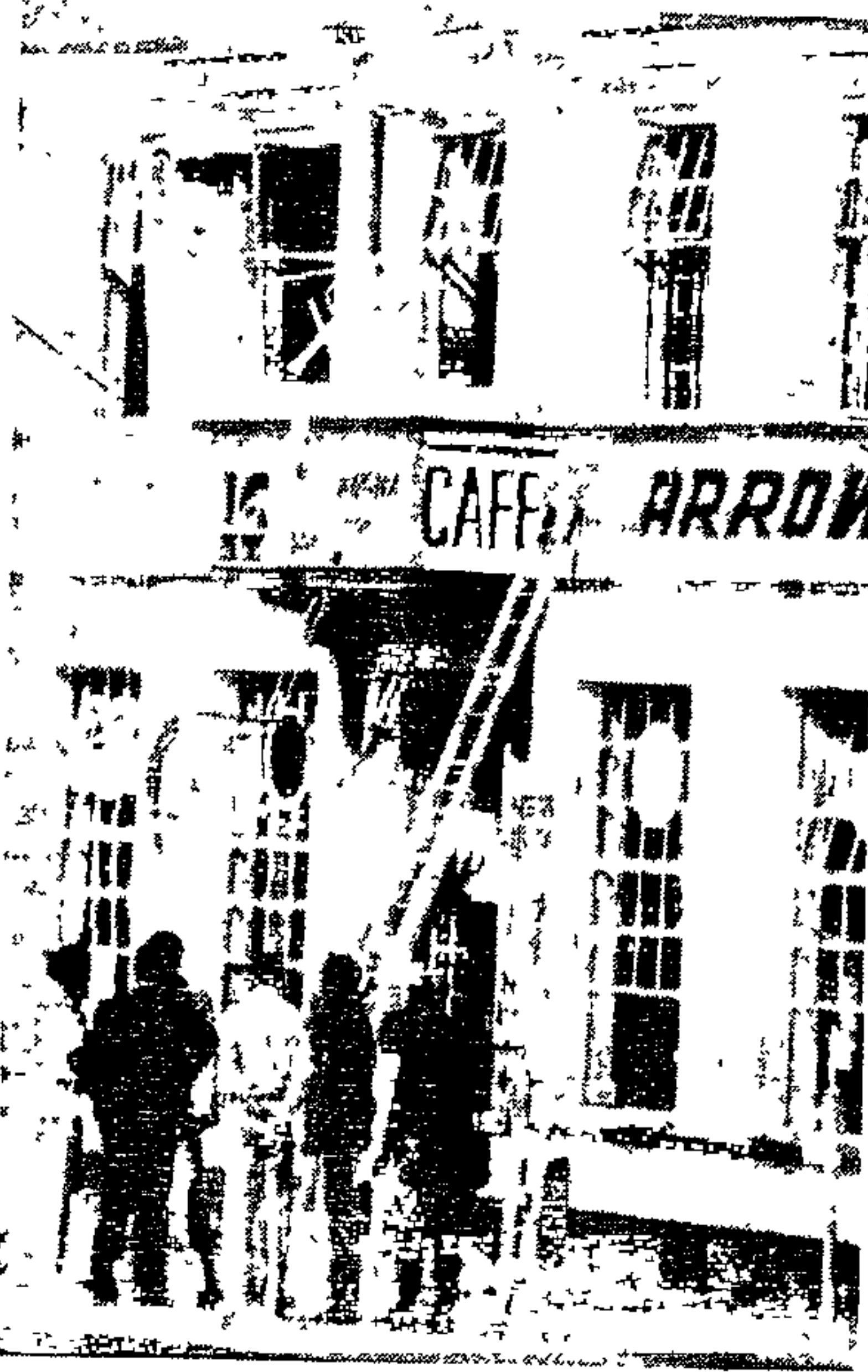
The building at 16 Angwa Street, Harare, after the SADF attack yesterday.
