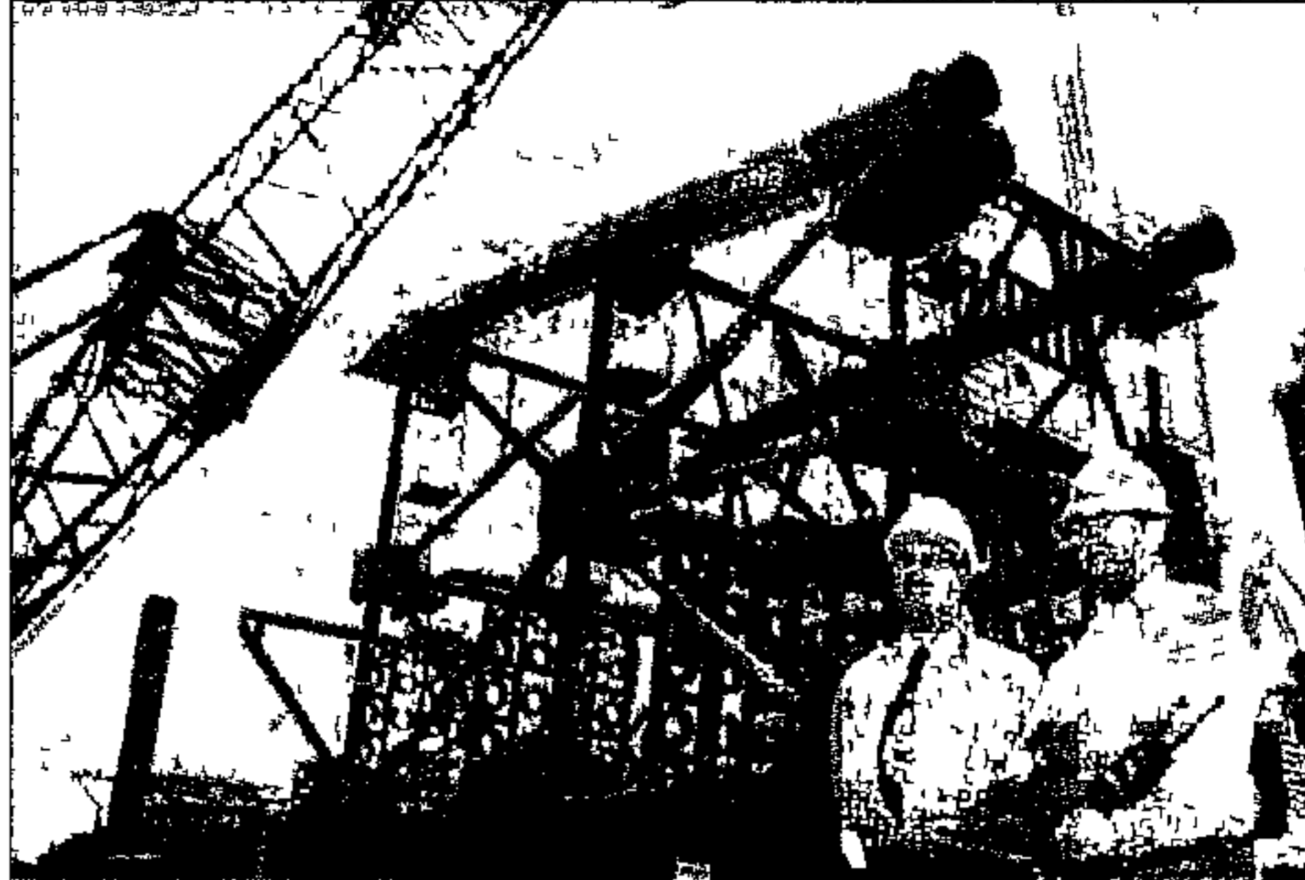
IN THE PIPELINE Further deals are on the cards, say John Cheeseborough and construction manager Eric Coull
