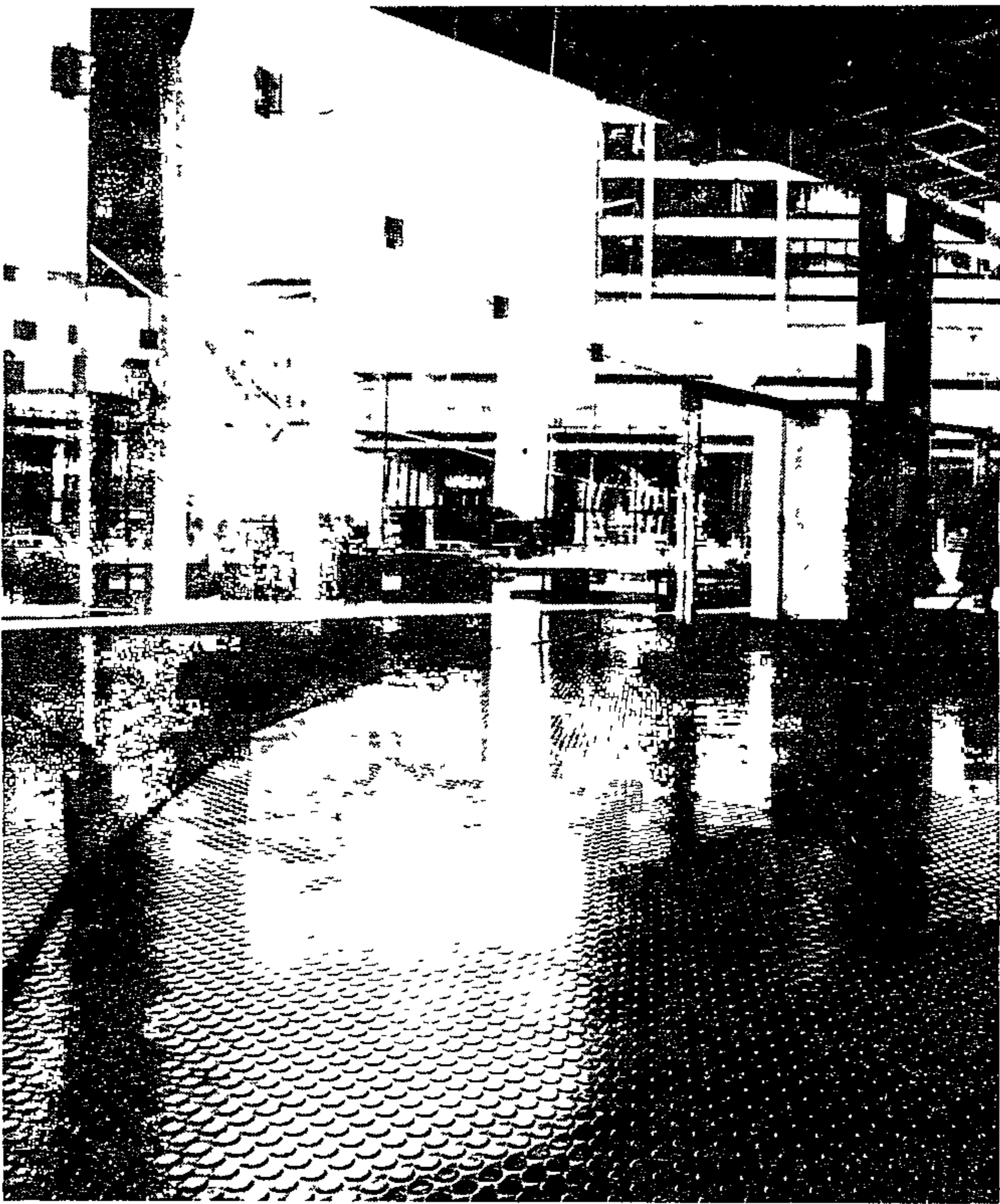
Toughened glass suspended from the ceiling hangs into a channel in the floor.
