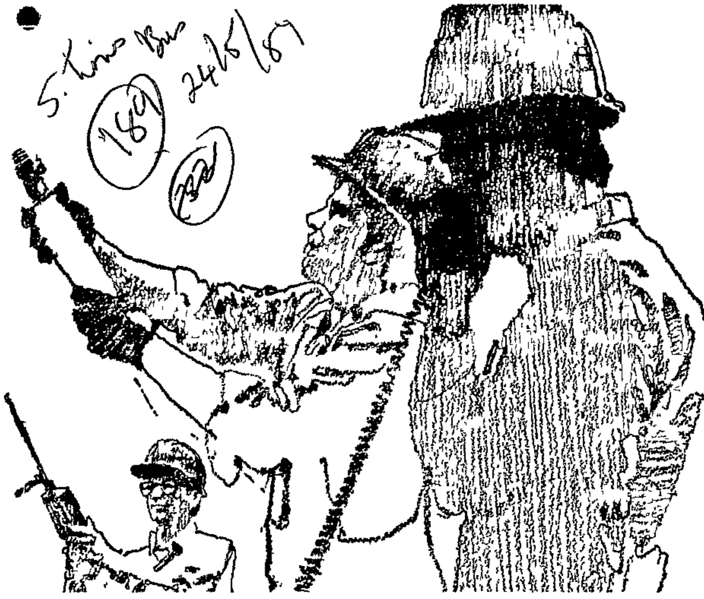
Construction workers . . . racing against time
