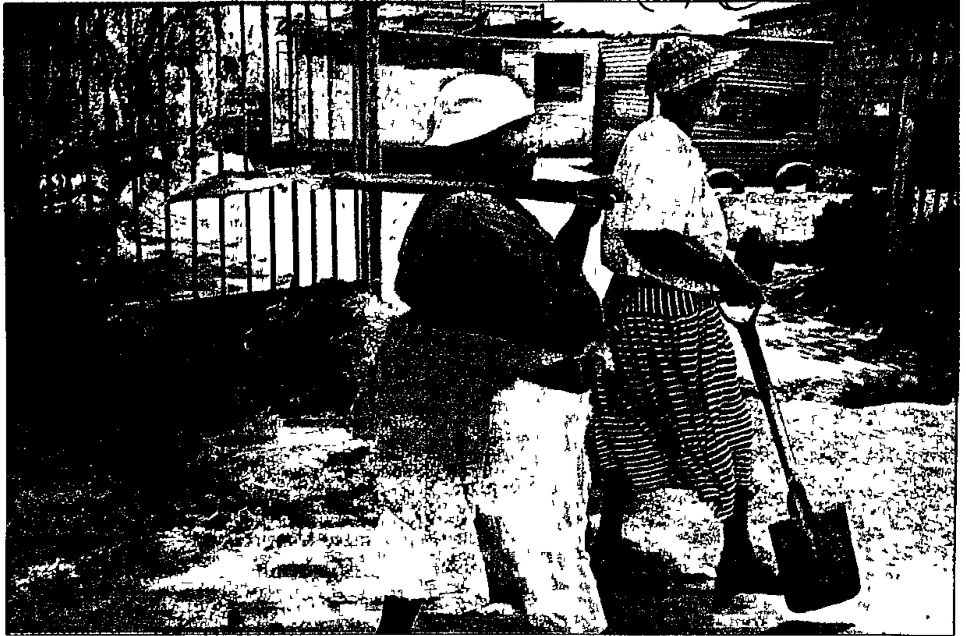
Now better protected ... workers on the way to dig trenches for street lights in Ivory Park.
