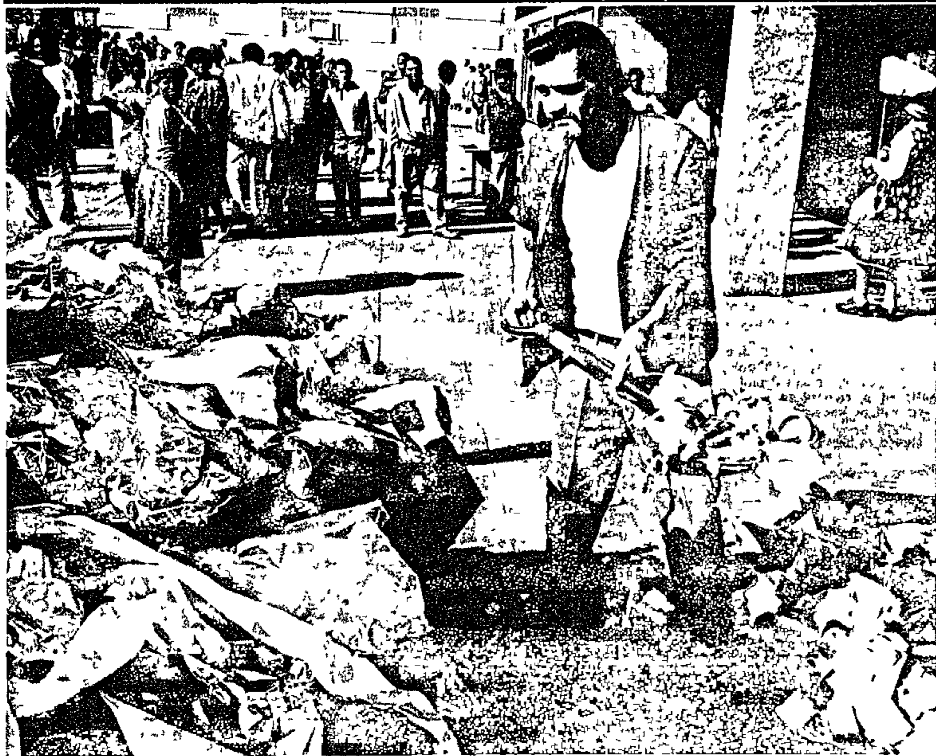
The railway workers' strike has left heaps of debris at central stations and some dirty employment opportunities, like this one at Johannesburg's Park Station
