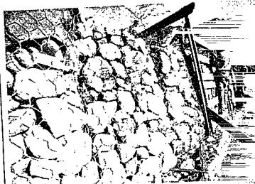
The wall in the new nursery extension Kirstenbosch Gardens, made from rows of wire baskets filled with stones.
