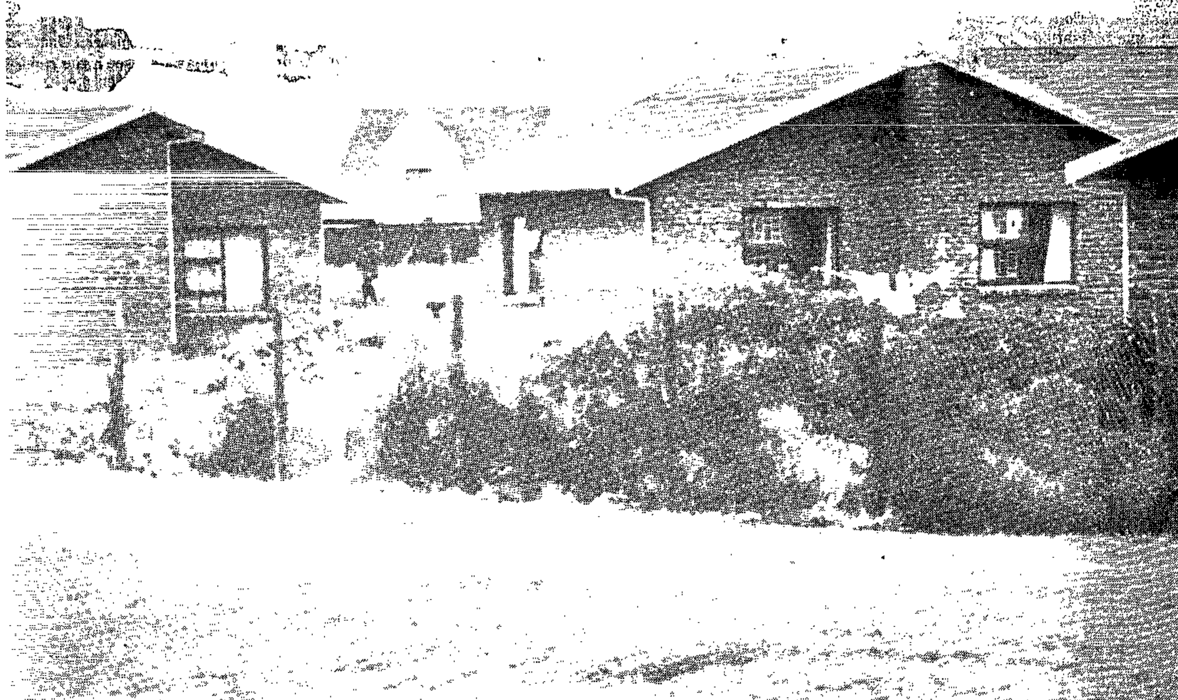
The row of houses for first-time homeowners built on the fringe of Bluewater Bay next to the N2 freeway — sites considered by some councillors and other residents to be an unfortunate choice for young couples.
