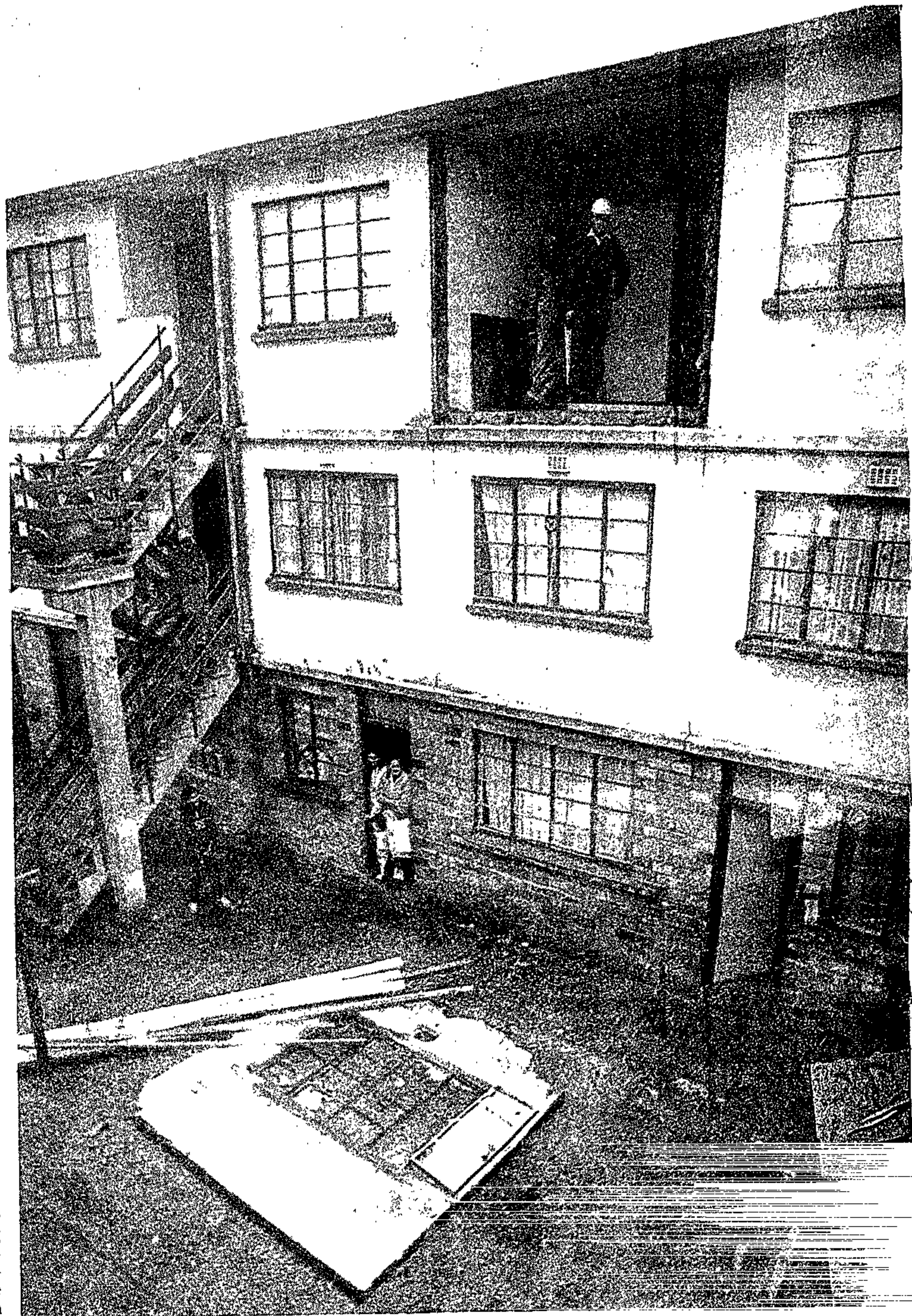
Residents of Irene Court in Heideveld gather in the courtyard as workmen from the Mechanical Engineering Branch of the City Council attempt to make temporary repairs to the flat. ● More weather pictures, pages 3 and 15 Picture: Ivor Markman
