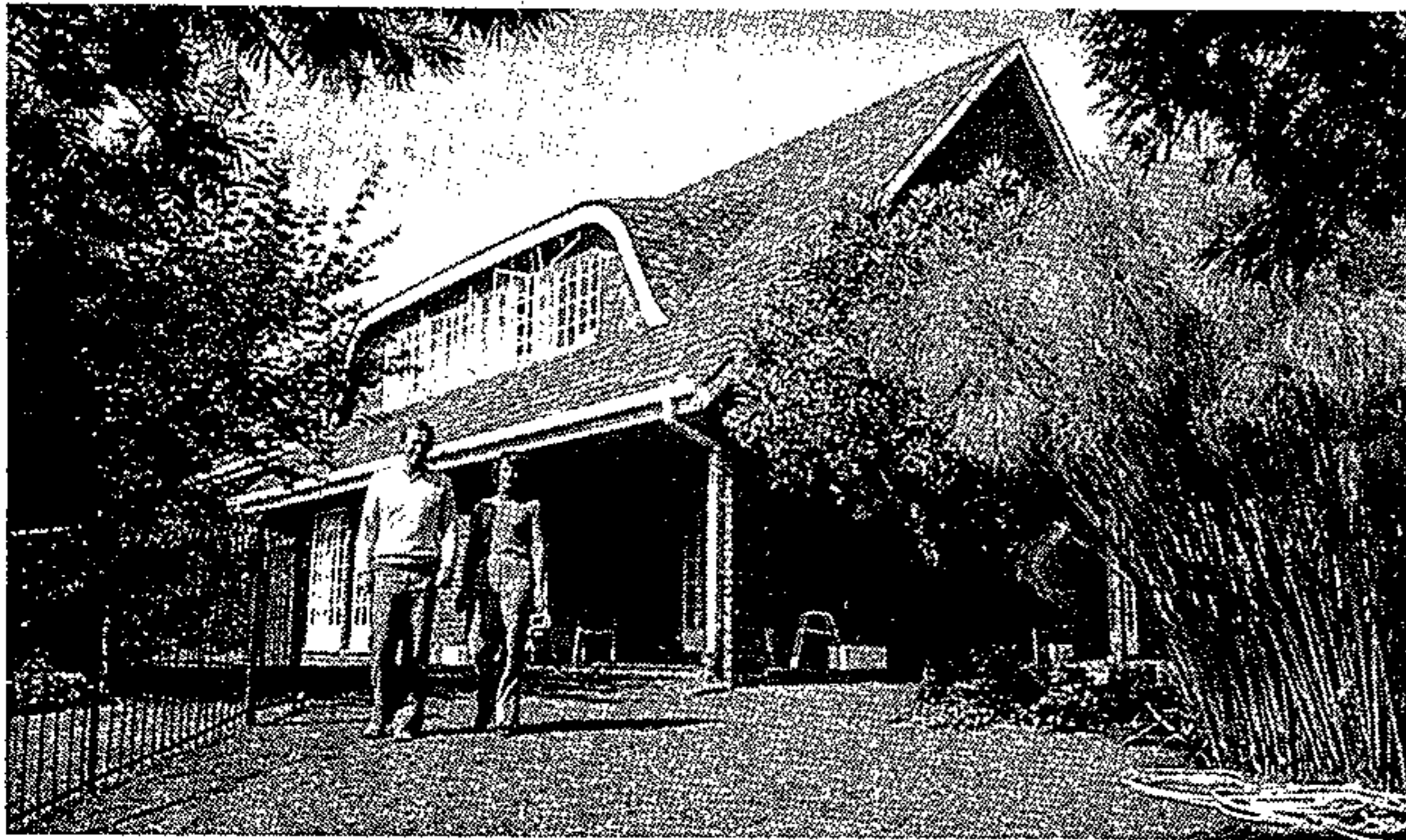
● From the outside it is impossible to tell whether a house is a timber-frame or conventionally built dwelling. This attractive house is timber-frame.
