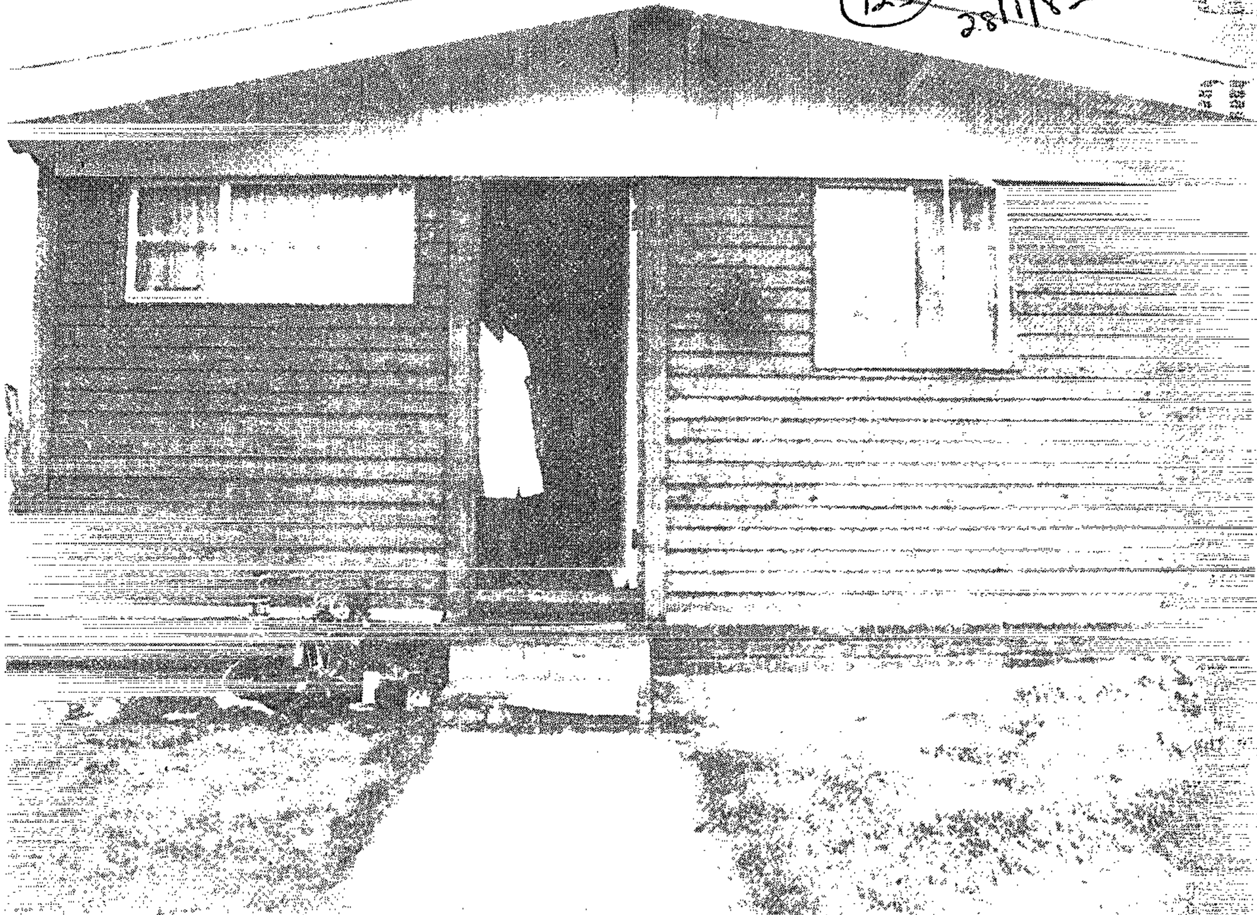
A log cabin-type home in Parkside which was built for R1 600 three years ago as a test project. According to the tenants, the house has required very little maintenance and is "very comfortable". It comes in kit form, complete with windows and roof.
