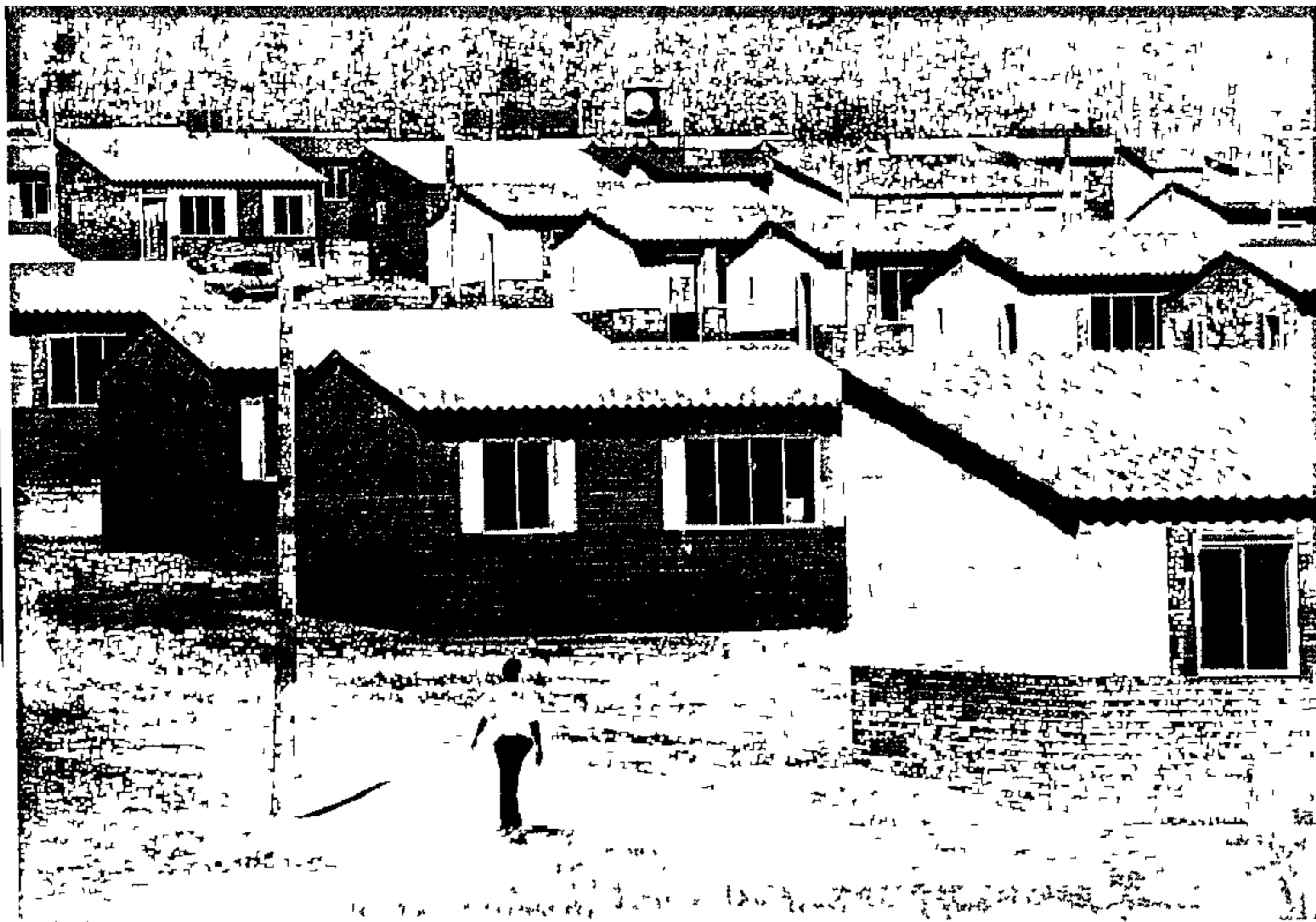
Construction of the 1 800 units making up the athletes' village for the All Africa Games in September is expected to be completed by the end of July. The village, which will house about 6 000 athletes, will be converted into low-cost housing when the games have run their course. Construction began in November last year. Picture: BRETT ELOFF
