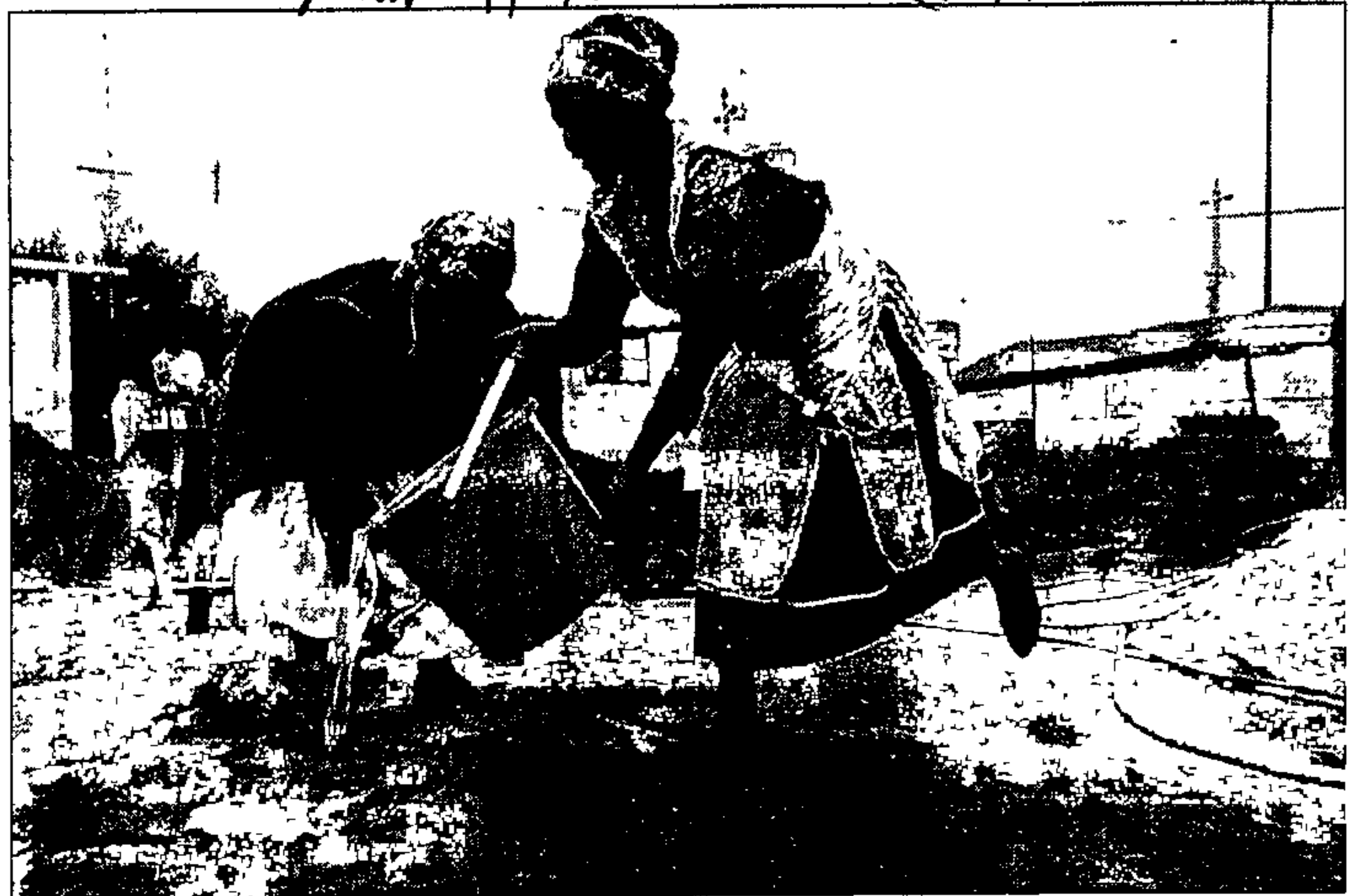
Joint responsibility ... women on the East Rand are building their own houses in a community self-help scheme.
