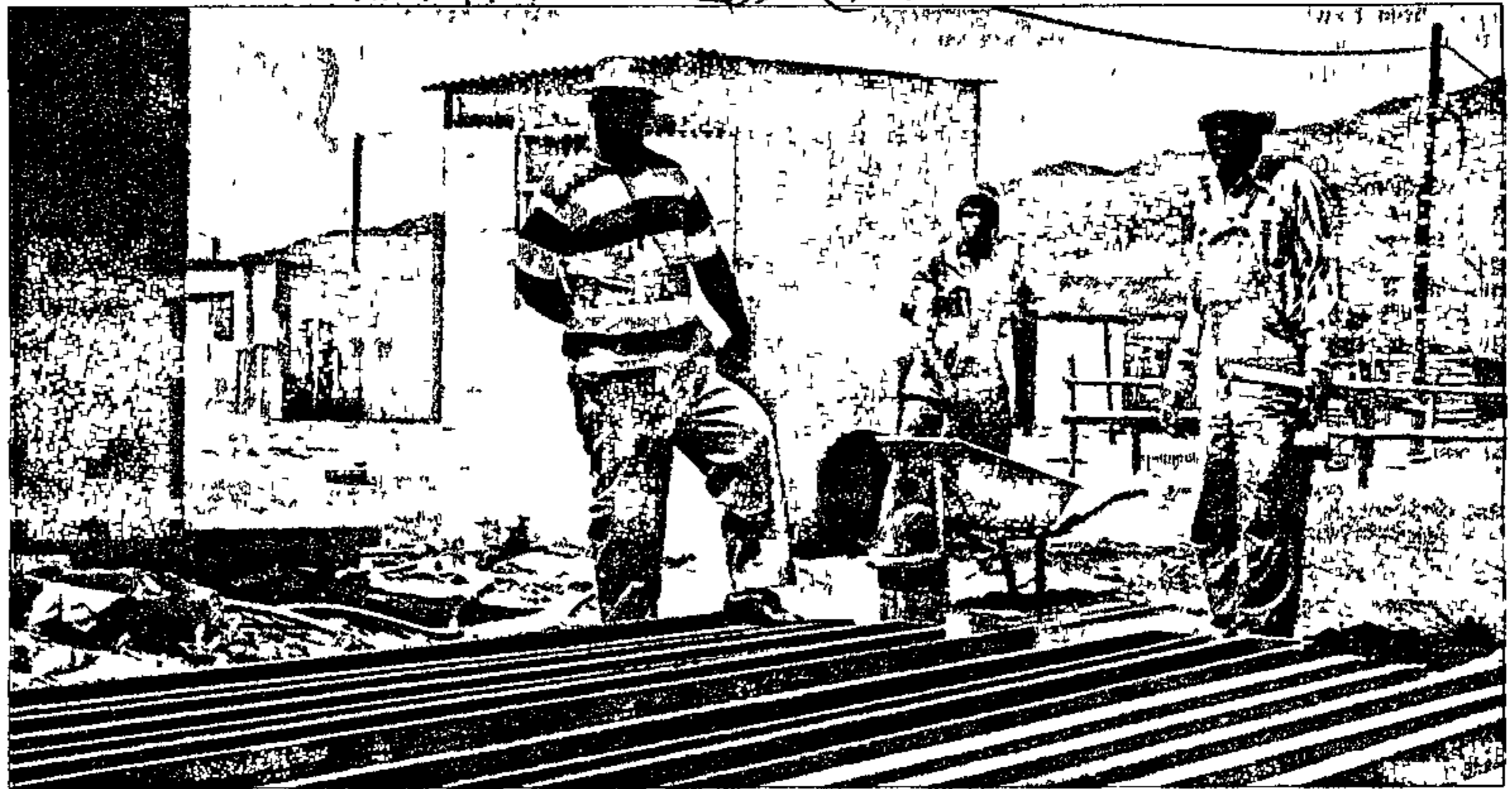
New start: Residents who can afford something better than a wooden shack are being helped by developers Communicare to build brick homes
