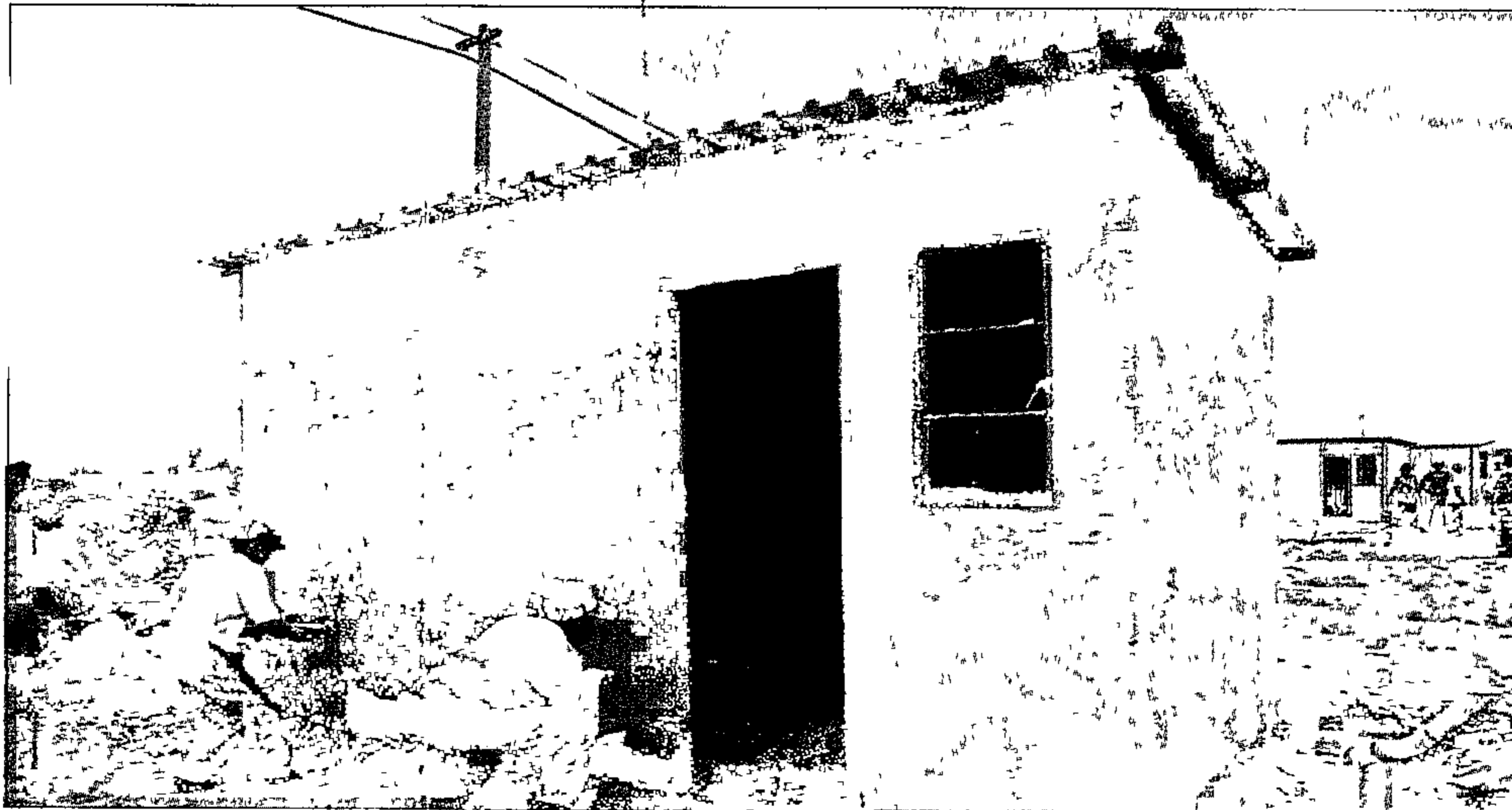
Home improvement: the houses are made of corrugated iron sheets and reinforced with foam rubber and wire mesh which is cemented and painted
