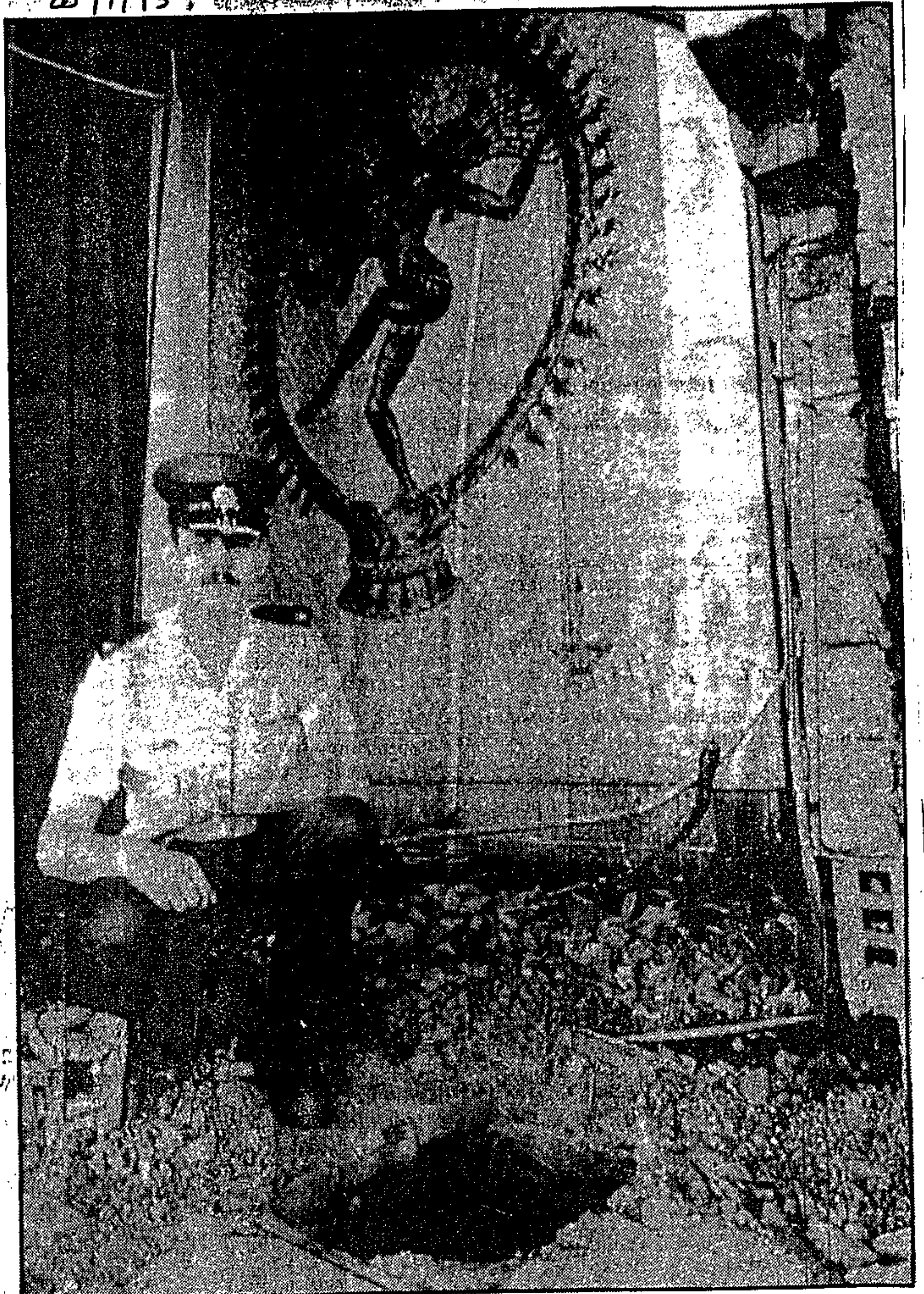
Damaged . . . Major Andrew Lesch inspects the Hindu temple in Laudium which was bombed early yesterday morning. Picture: John Hrusa
