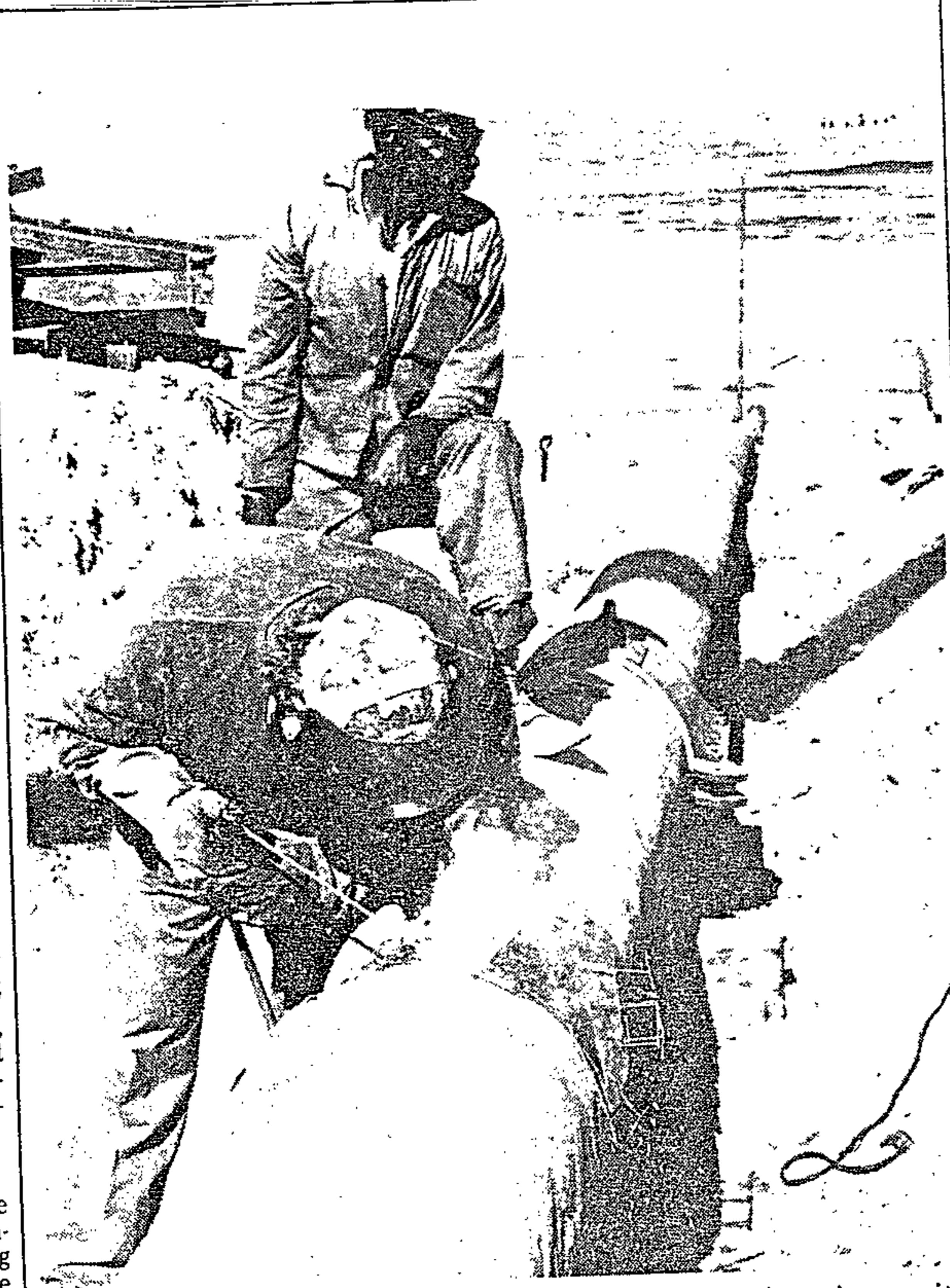
WORKMEN complete the final weld on the steel and gunnite protective sleeve which will house the plastic pipe.
