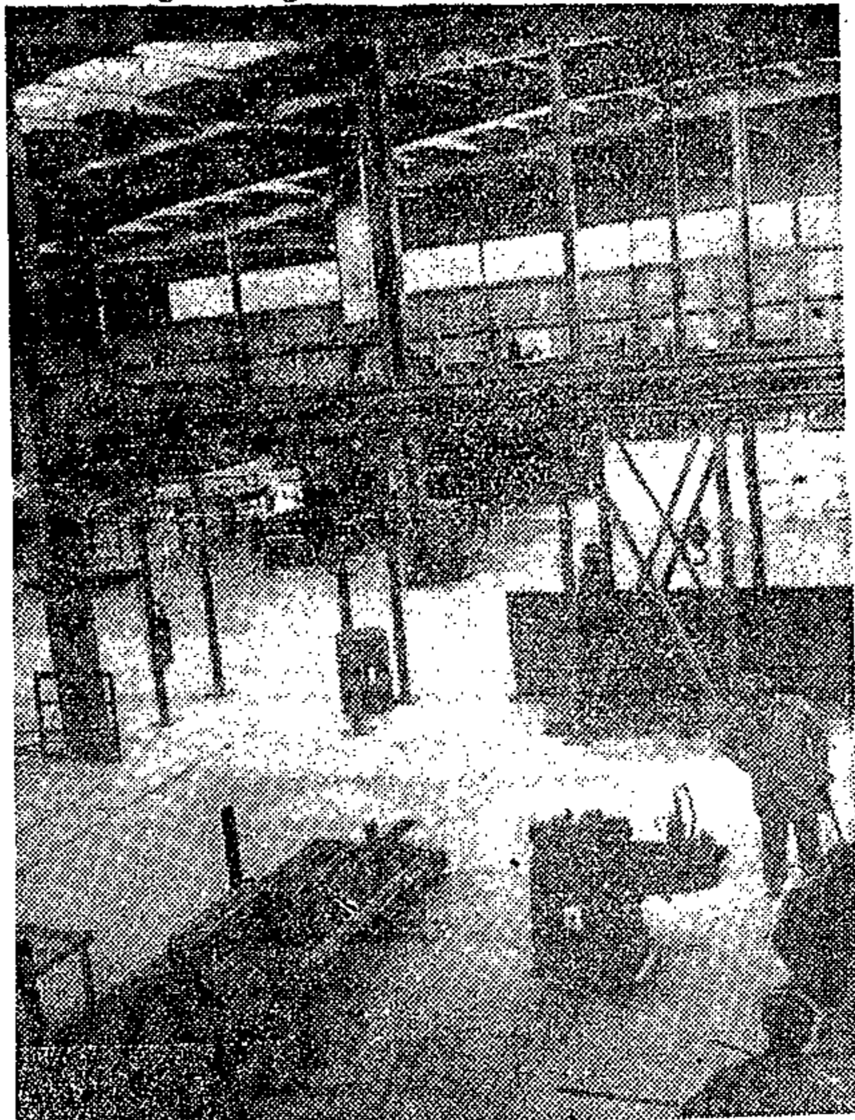
A general view inside the Wispeco factory which was opened yesterday by the Minister of Bantu Administration, Mr M. C. Botha.
