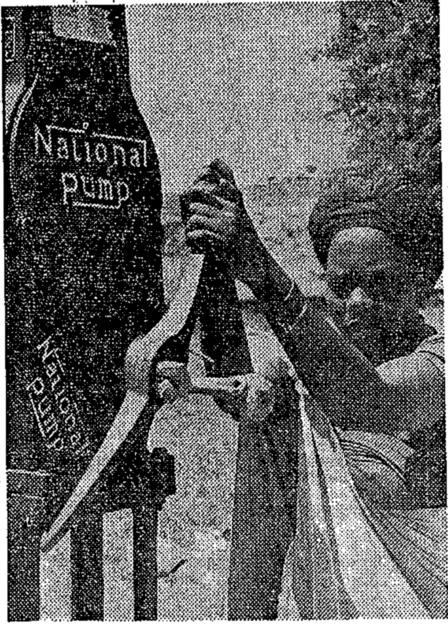
Using a bit of ingenuity, a woman fits a pickaxe handle to a vandalised borehole and draws water
