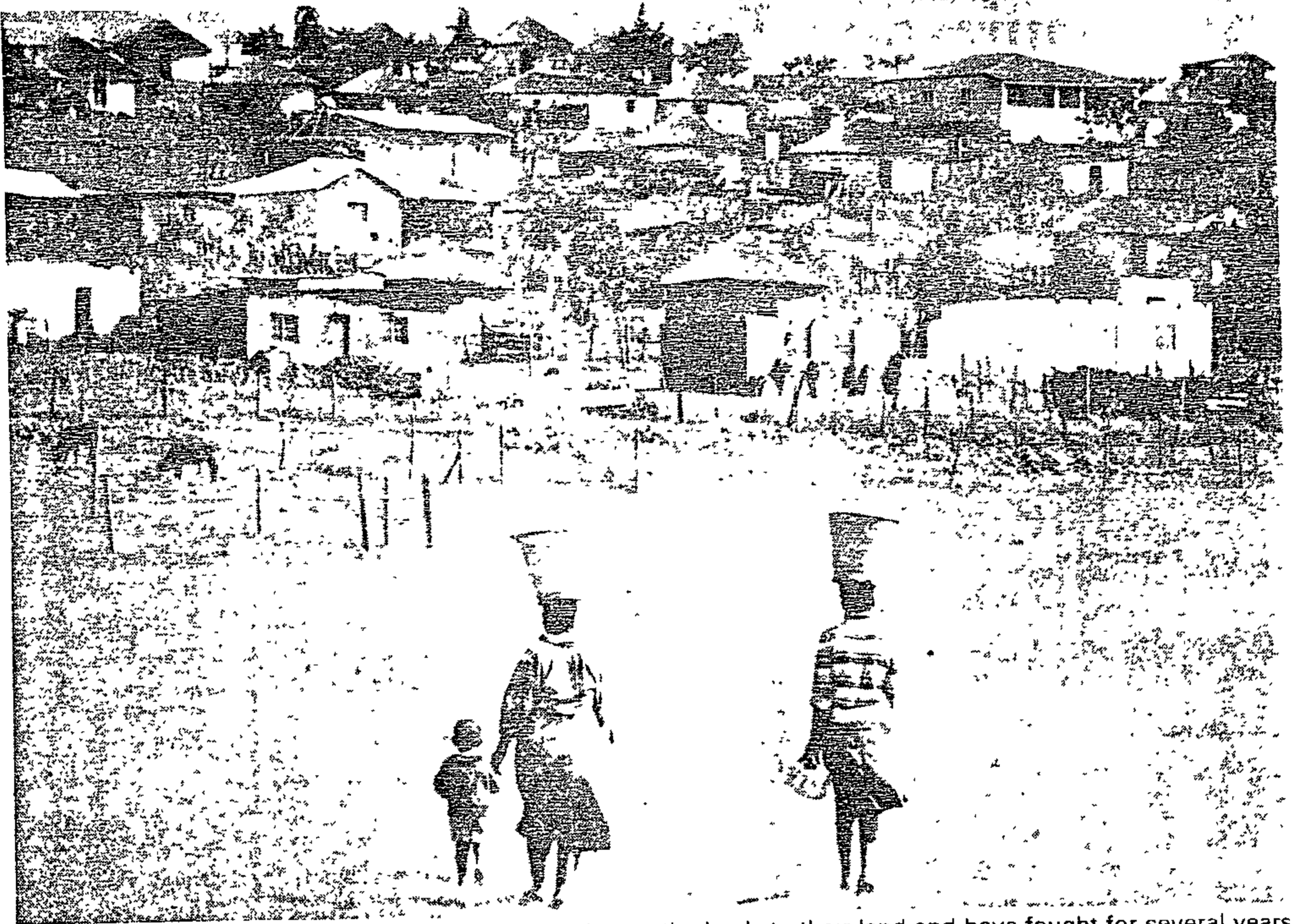
Mgwali village where many of the householders have title deeds to their land and have fought for several years to be allowed to stay.
