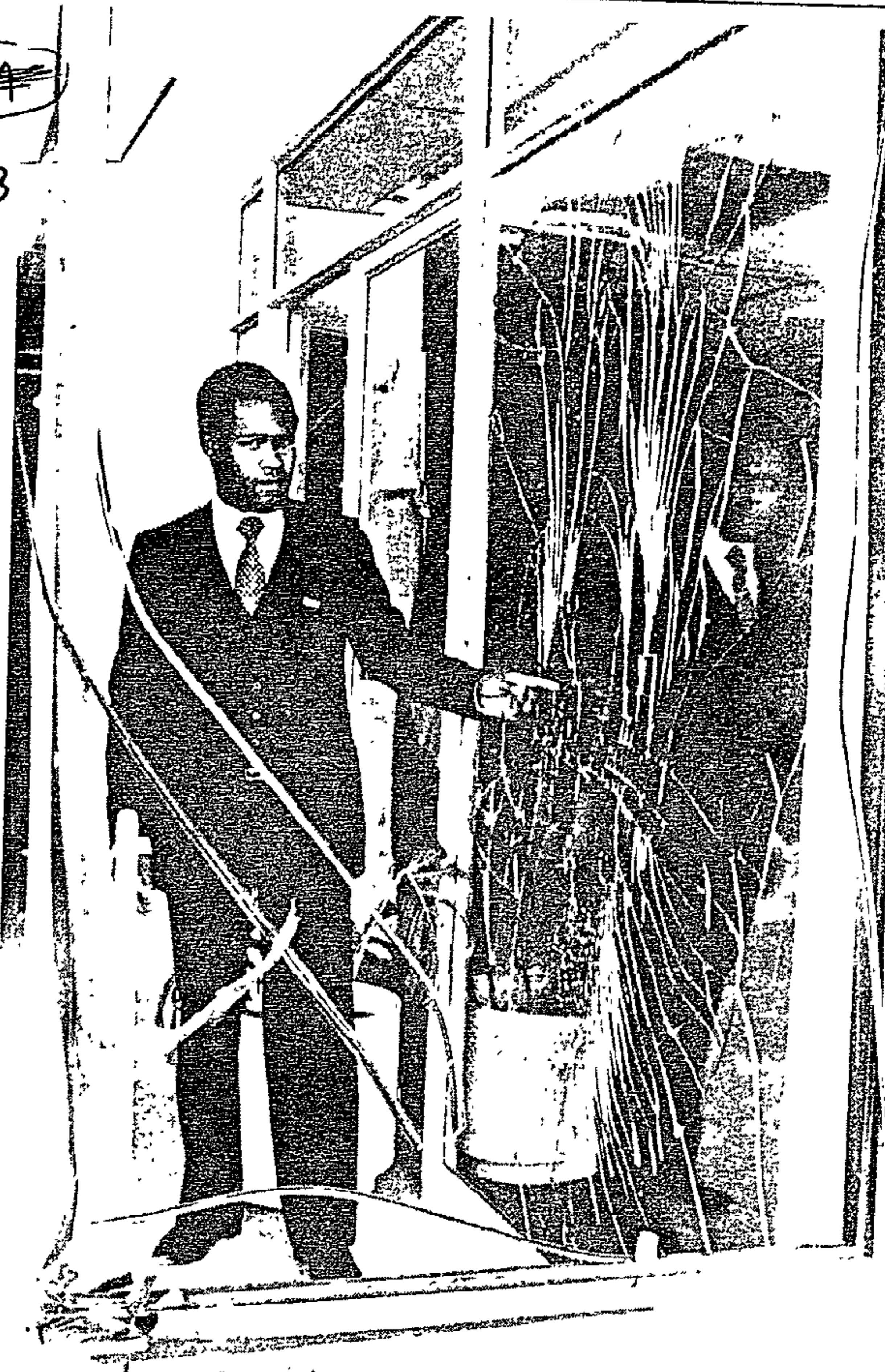
Mr Thobile Mda, a ministerial counsellor, points out some of the damage caused to the Ciskeian Embassy by a limpet mine blast on Sunday night.
