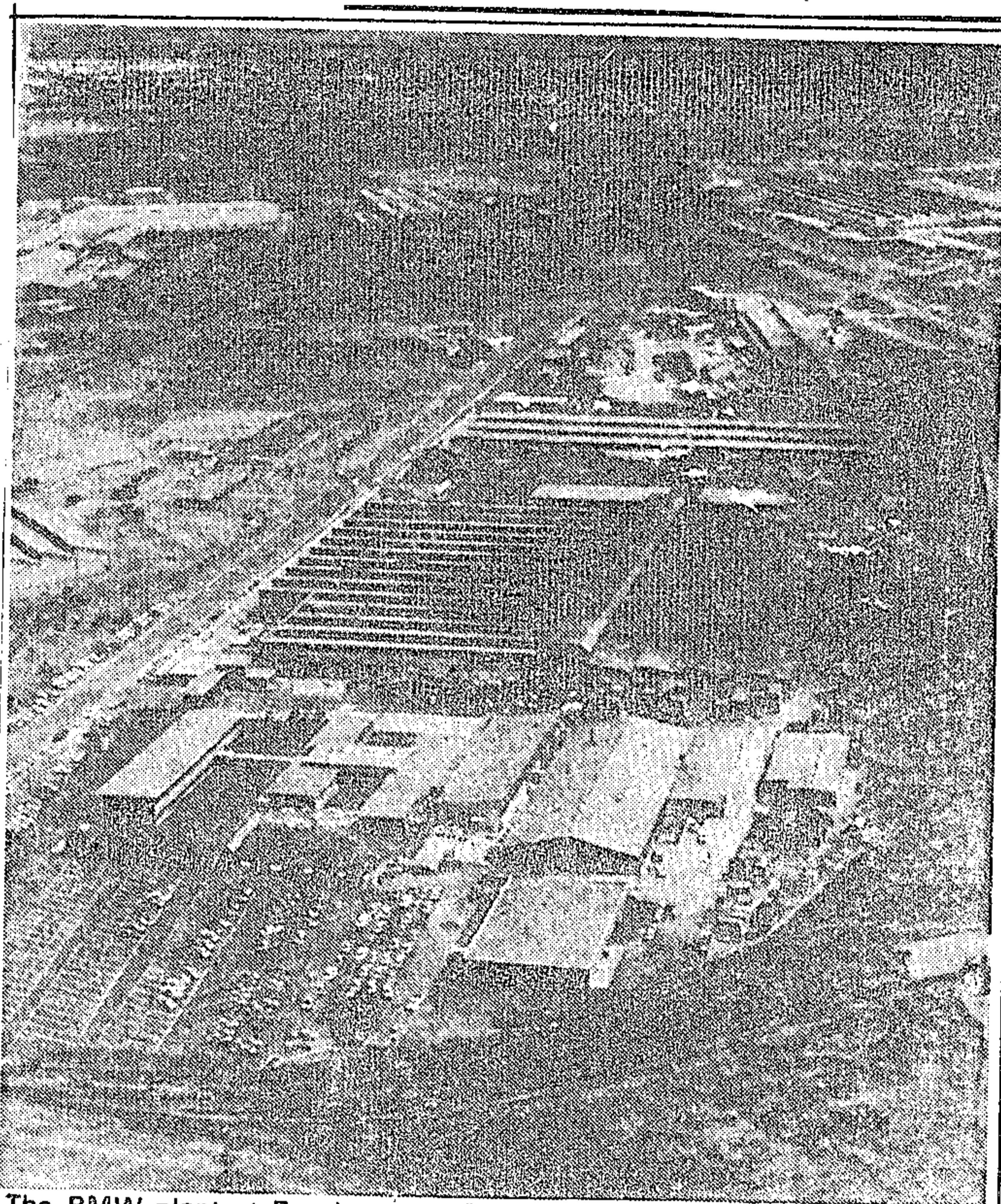
The BMW plant at Rosslyn, near Pretoria, which is to be extended at a cost of R52-million. The extra capacity is scheduled to come on stream in mid-1983.
