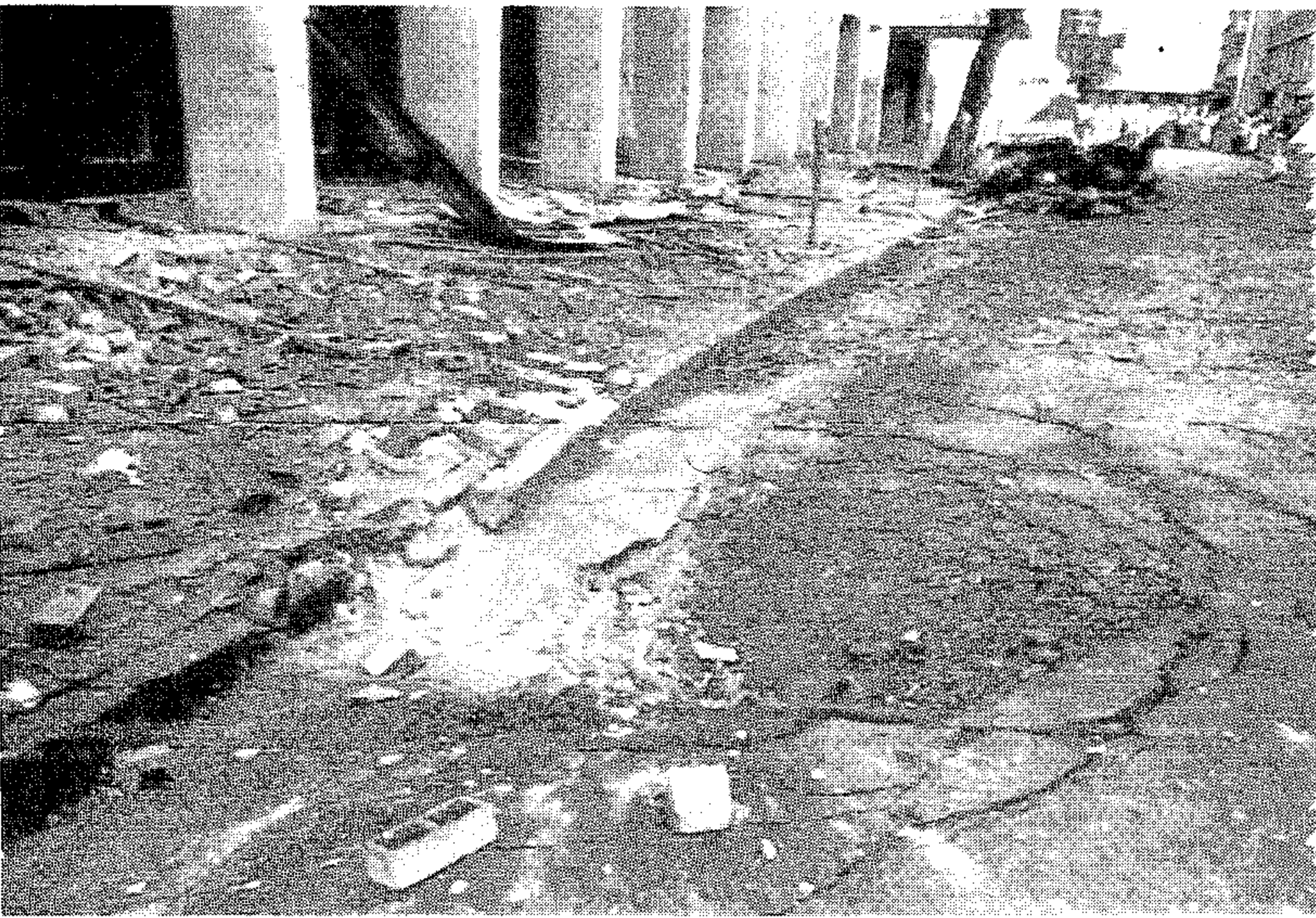
The hole left in the road by the impact of the blast.
