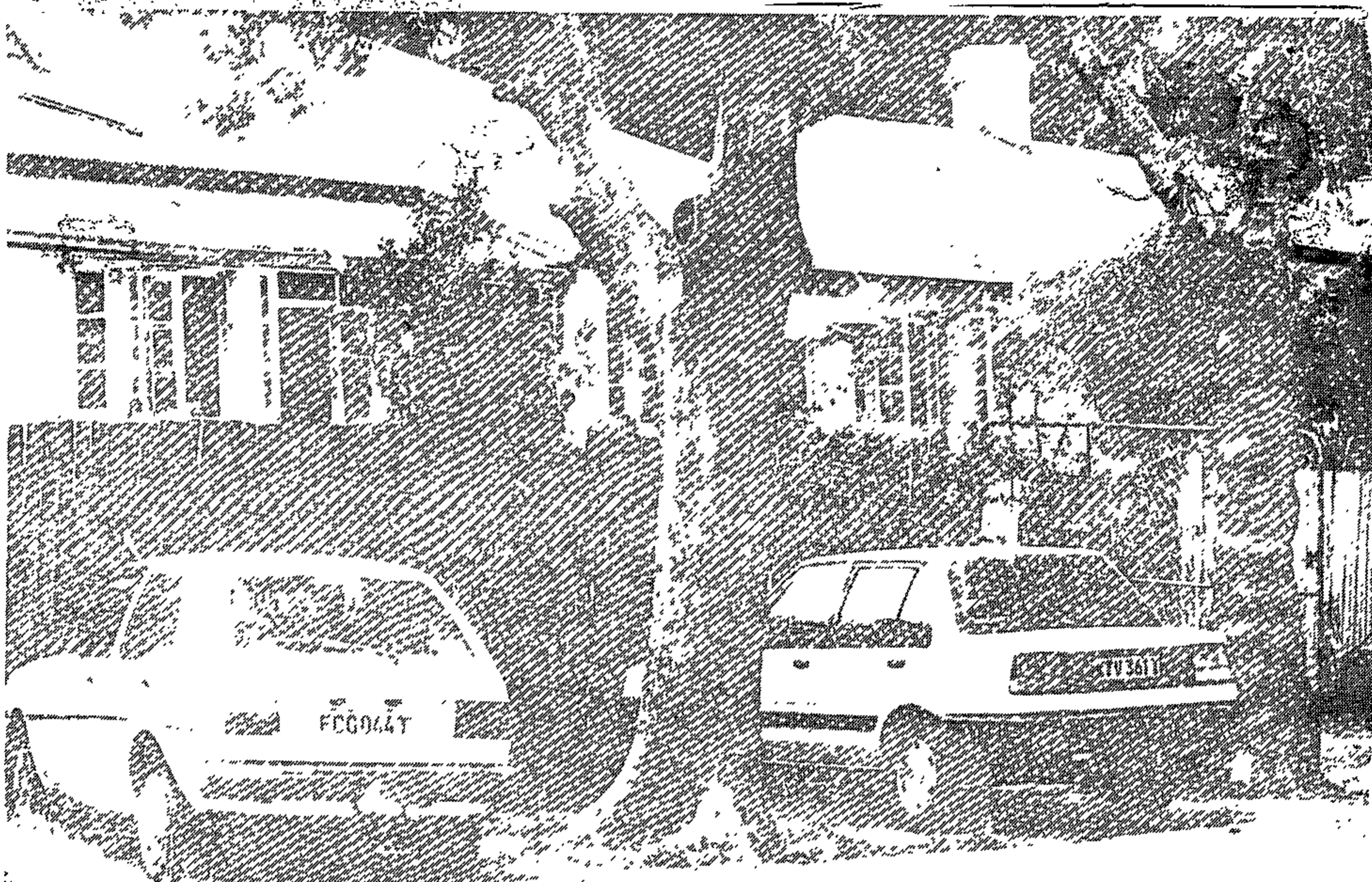
SOME of the houses at Laanglaagte Deep (also known as Crown Mines) which are to be closed down this month.
