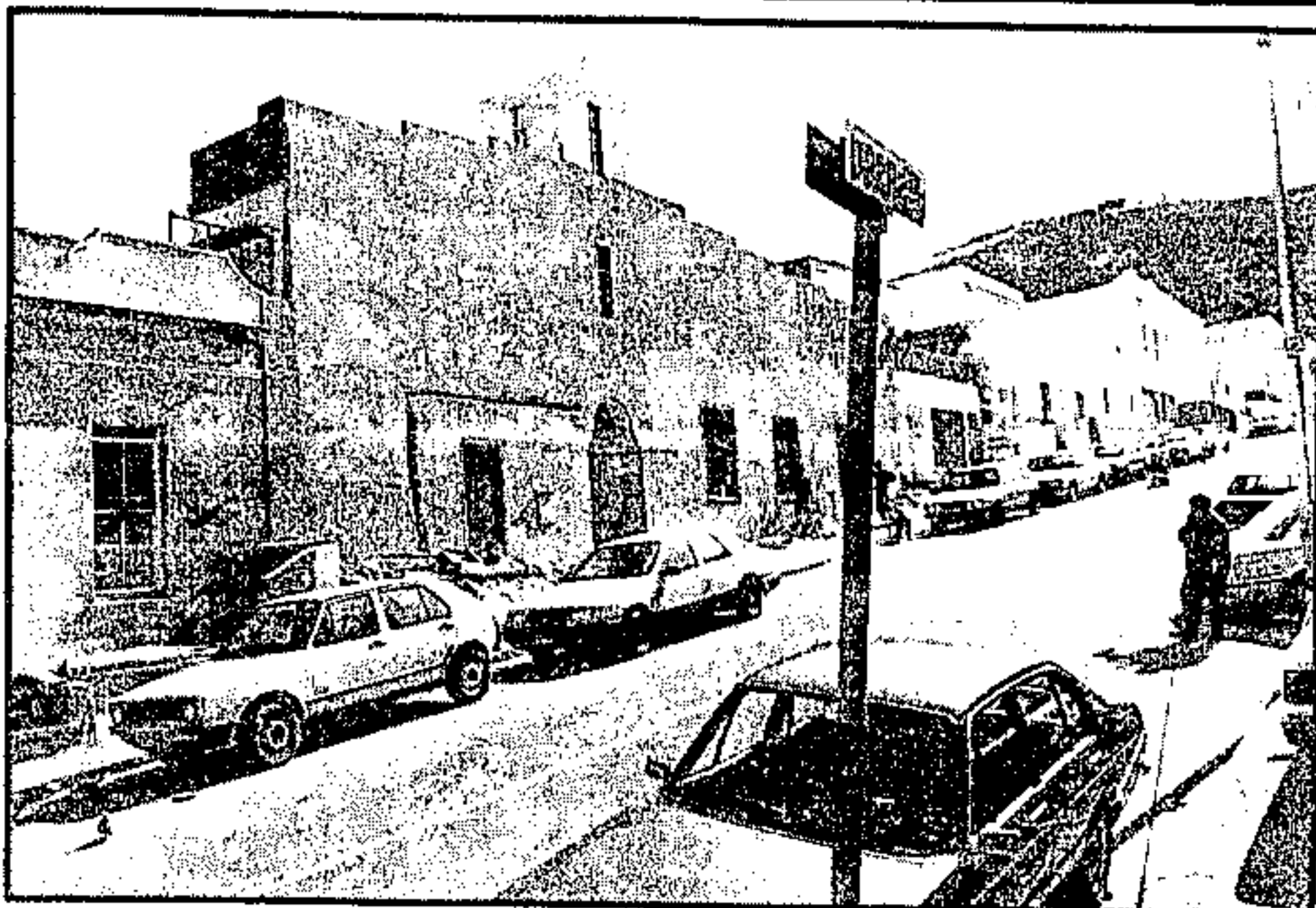
NEEDS REPAIR: The Engol family home for 34 years. It requires almost R80 000 for renovation
