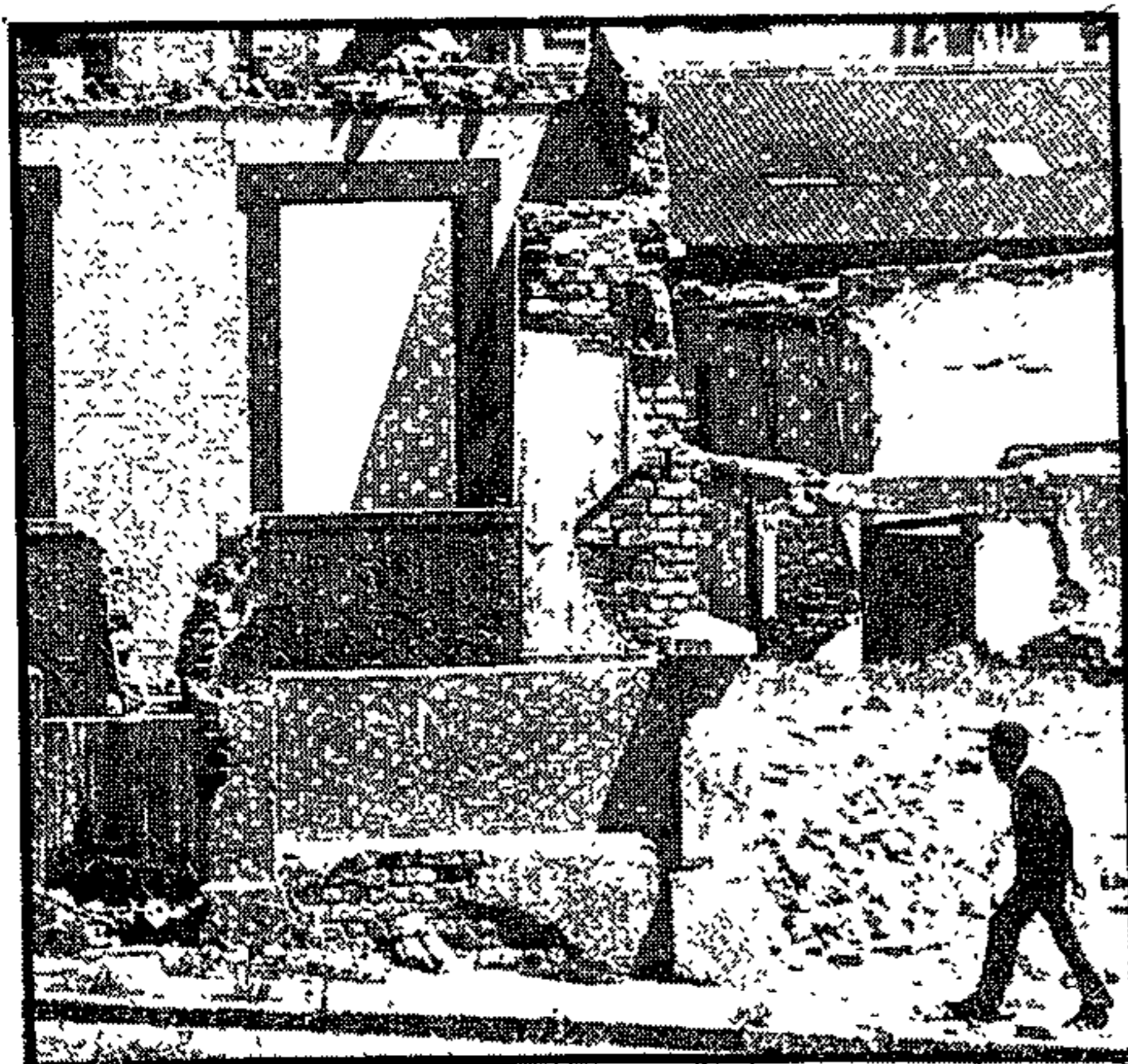
A crumbling world: remains of homes in the process of demolition.
