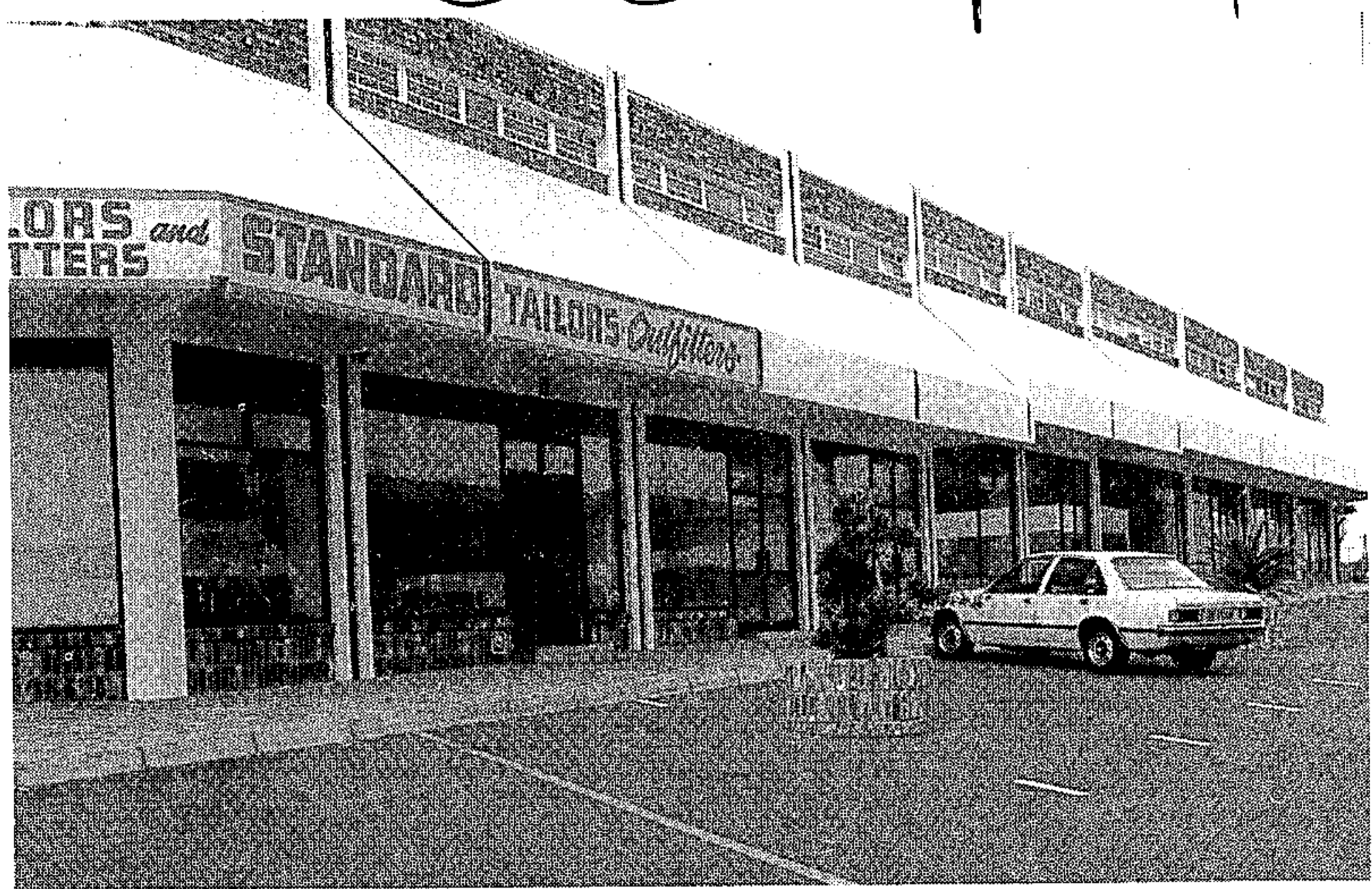
Shops at the Oriental Plaza. Those on the right are unoccupied.
