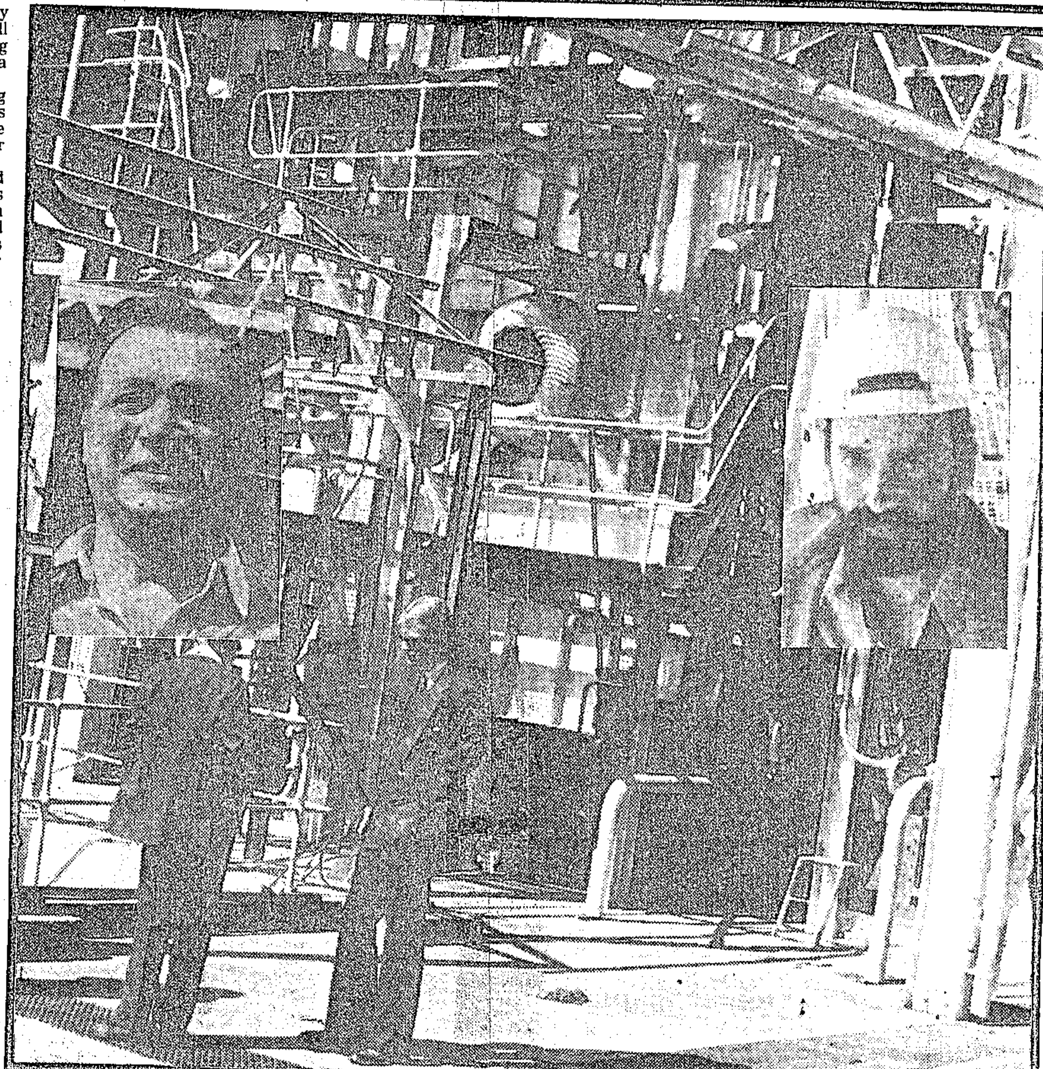
Part of the old Tzaneen power station, which will produce "dirt cheap" steam for the company's production plant. Insets show SAEF's chief backer, Mr Ken Buckerfield, left, and his partner, Mr Ken Ottignon.
