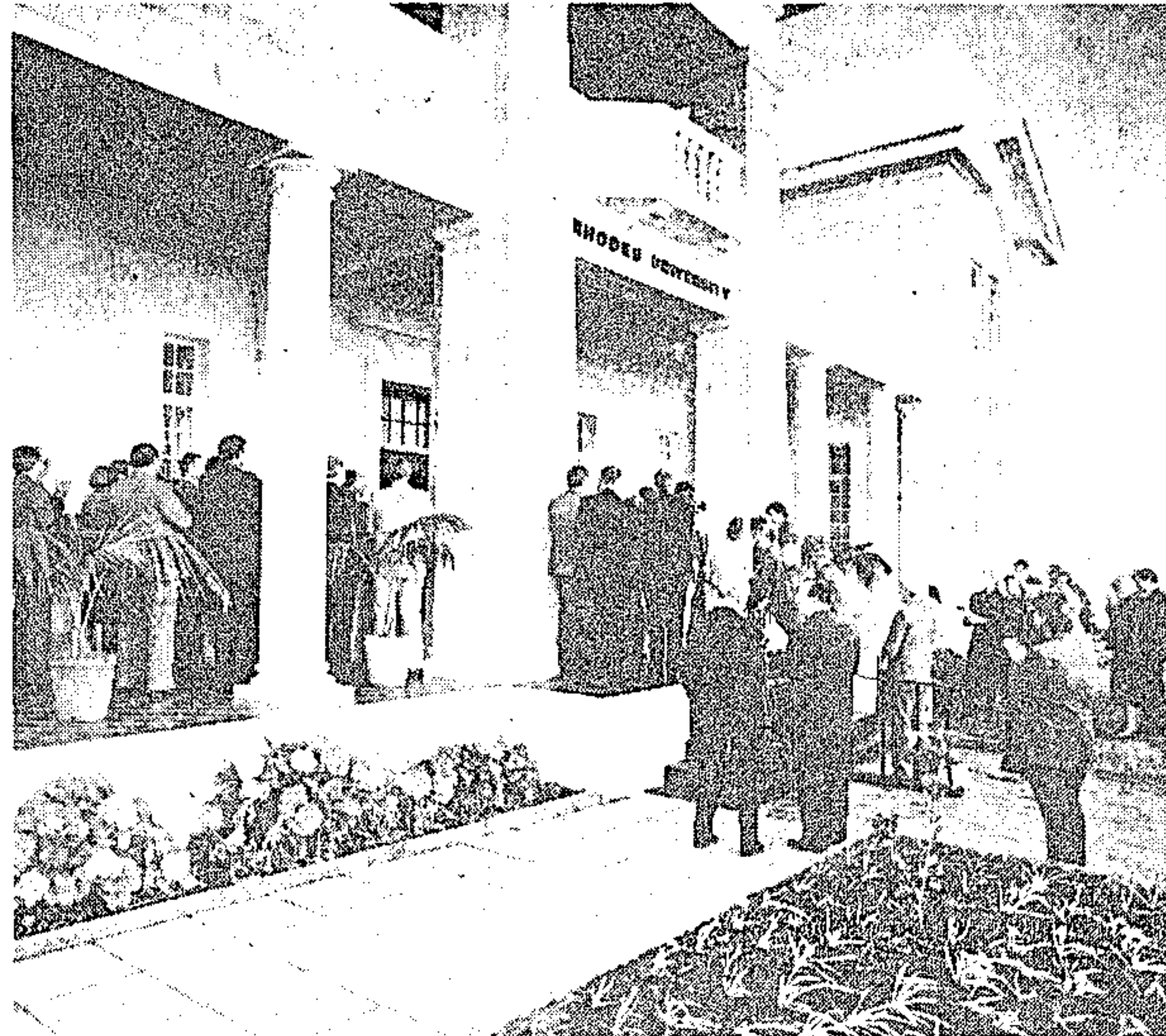
Honoured guests and Rhodes University officials gathered round the terrace of the old Wool Exchange building, now home to Rhodes University, East London, in Church Street yesterday to witness the unveiling of a plaque by the Chancellor, Dr Ian Mackenzie, declaring the building a national monument.
