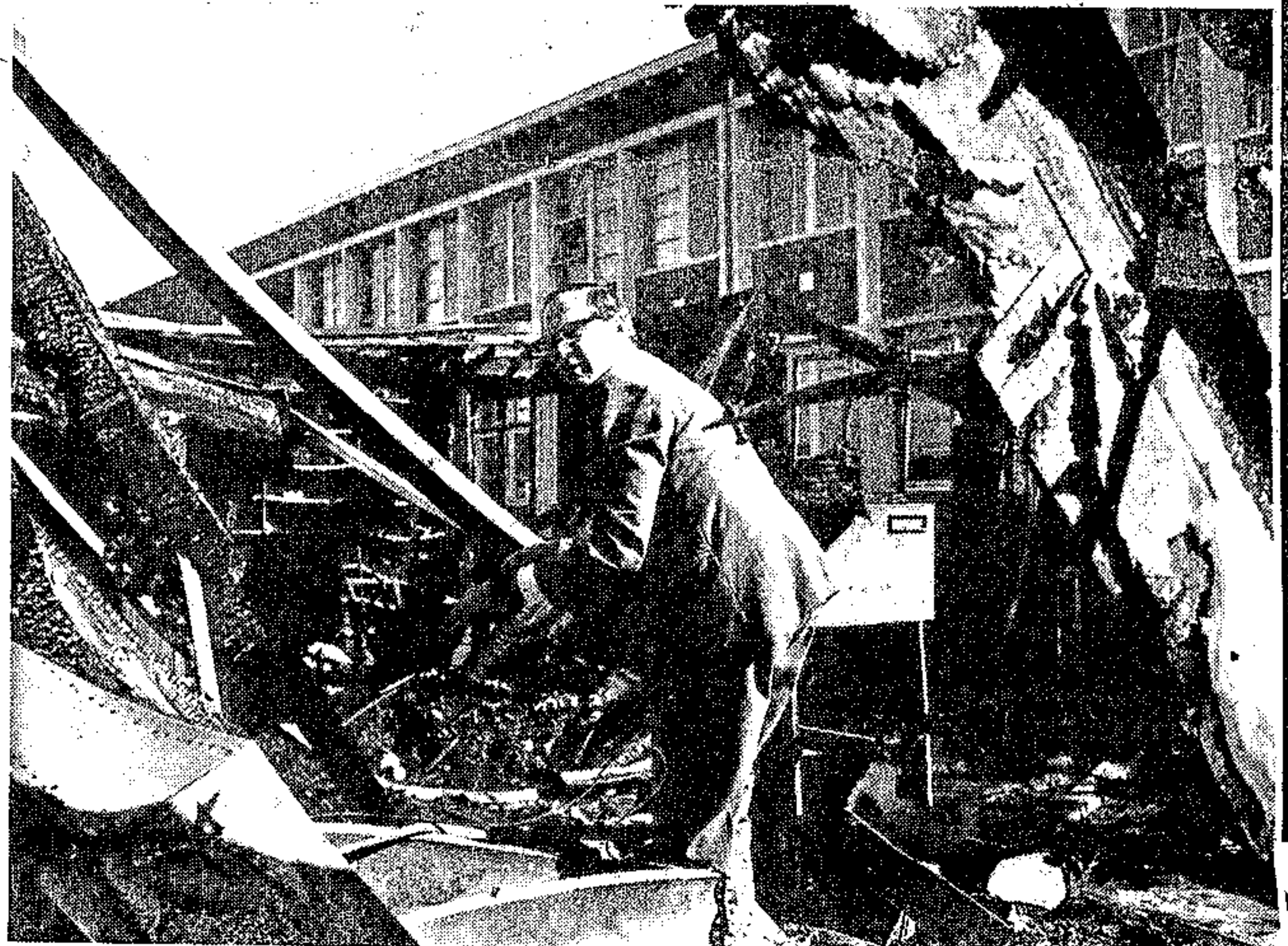
Part of the building that was destroyed at the university.
